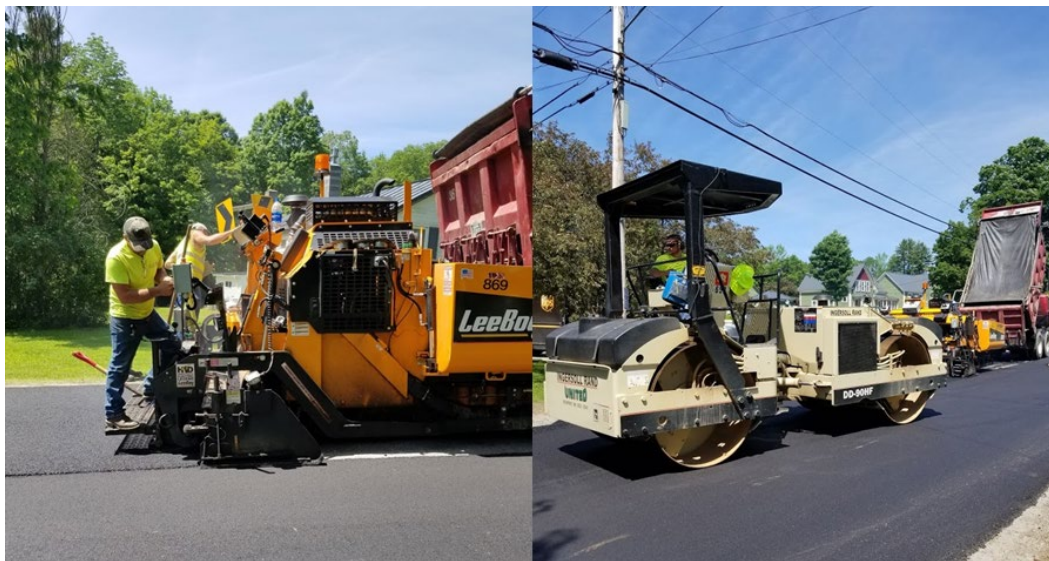
Figure 13. Test section construction on Corbin Road.
