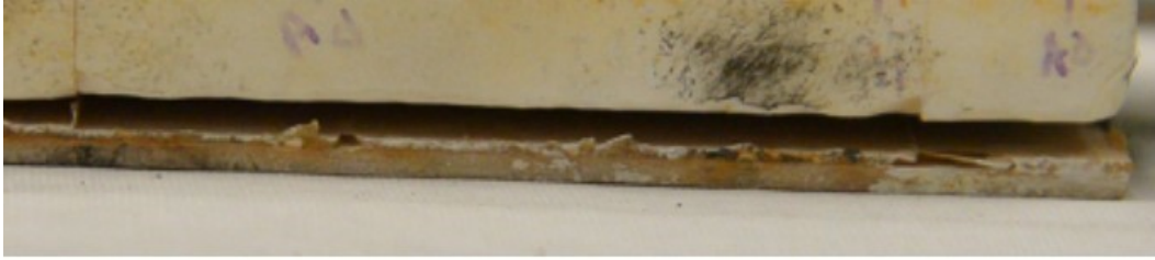
Fig. 19 Adhesive failure at the ceramic–composite interface due to ambient environmental exposure
