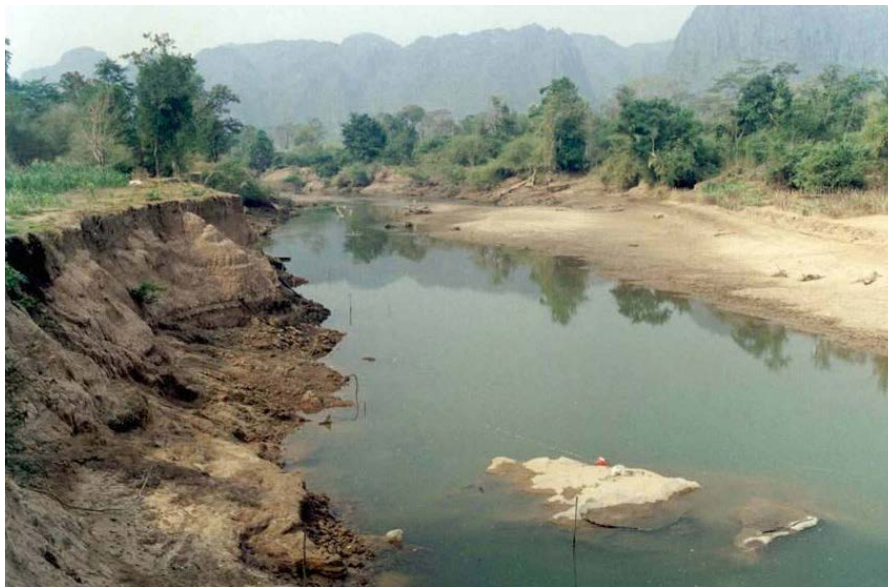
Figure 15. Erosion downstream of the Nam Theun-Hinboun Dam due to hydro-peaking of flows 119
