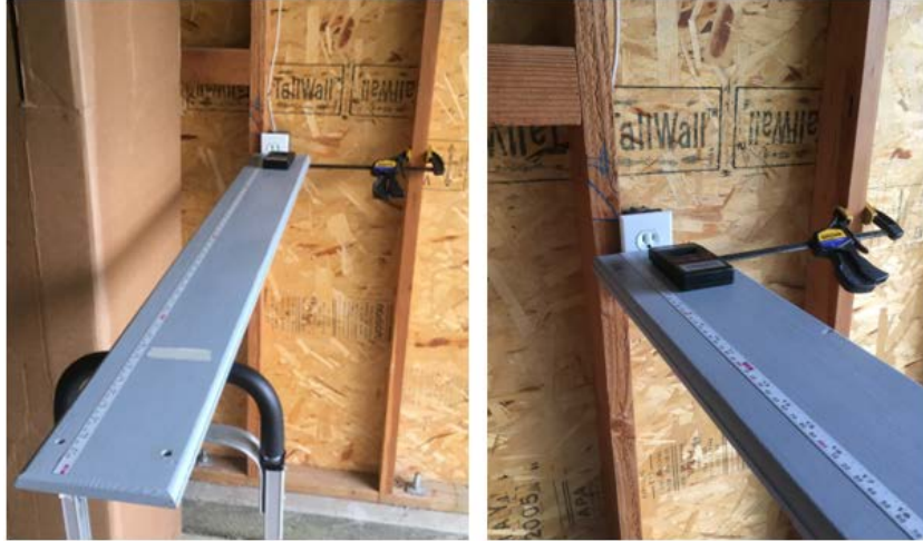
Figure 8. Testing Apparatus for 110V System
