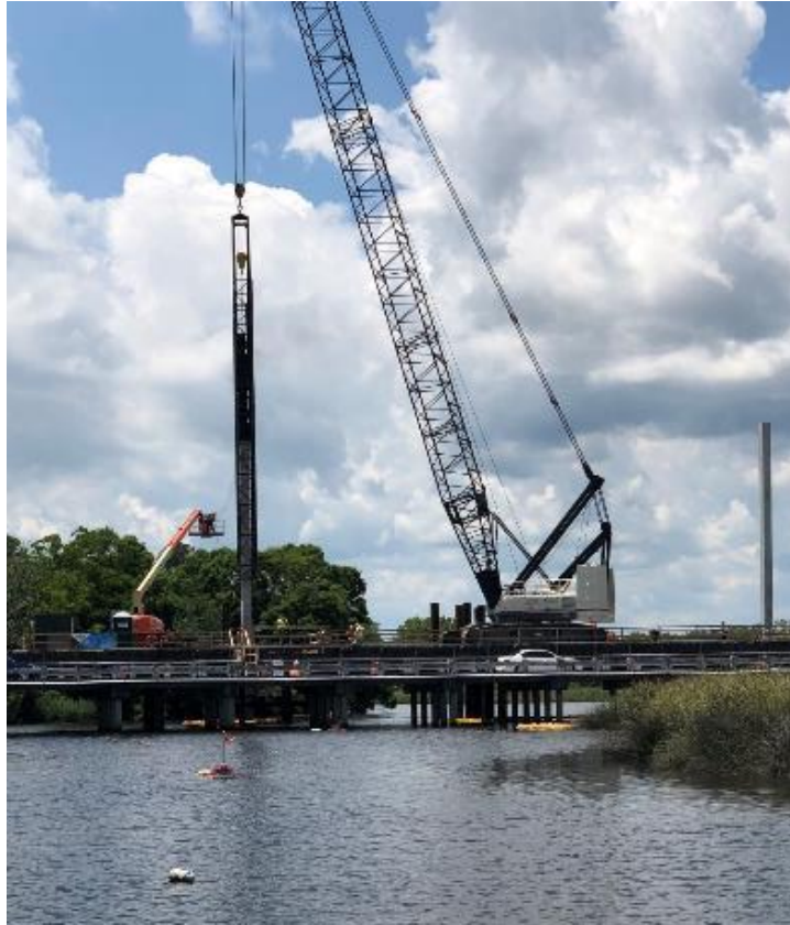
Figure 4-6. Pile driving at Ribault River (May 7, 2019 test pile shown)
