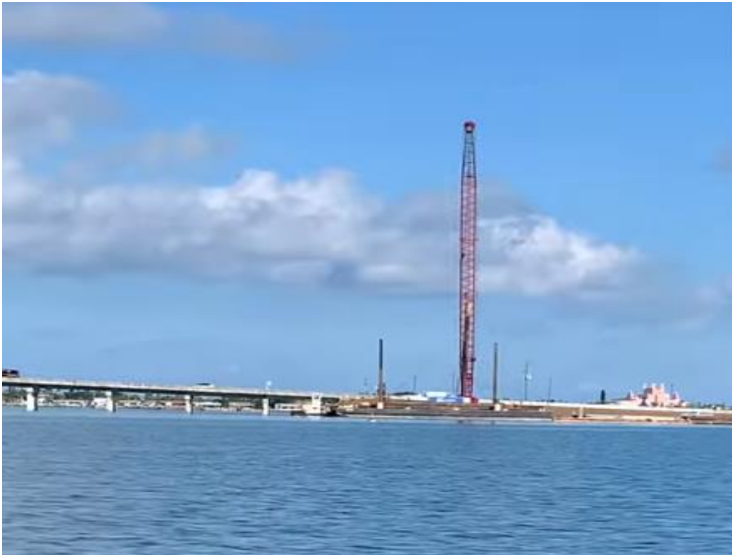
Figure 4-16. Pile driving at Bayway E Bridge on June 4, 2019.
