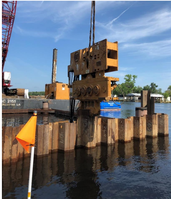
Figure 4-2. Vibrating hammer and sheet pile cofferdam at Dunn’s Creek
