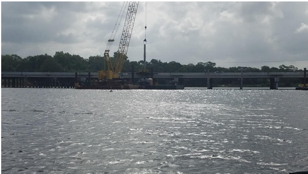
Figure 4-20. Concrete pile being placed into position at John Sims Parkway Bridge
