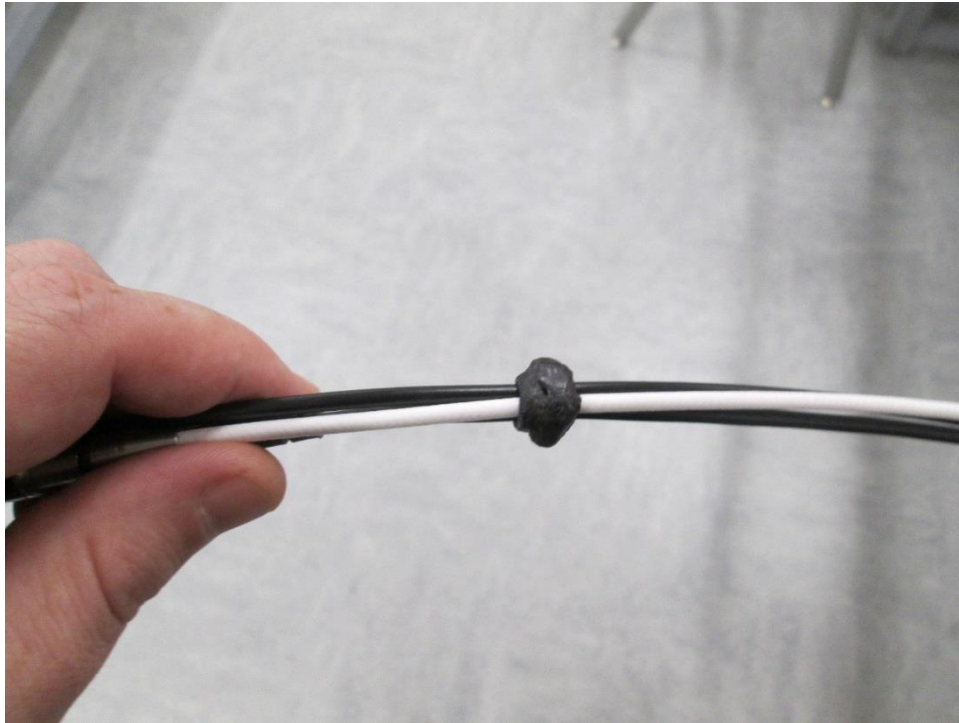
Figure 2-4. Cinch knot used to join the cables.
