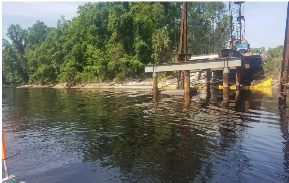
Figure 4-12. Steel trestle piles driven at Suwannee River Bridge
