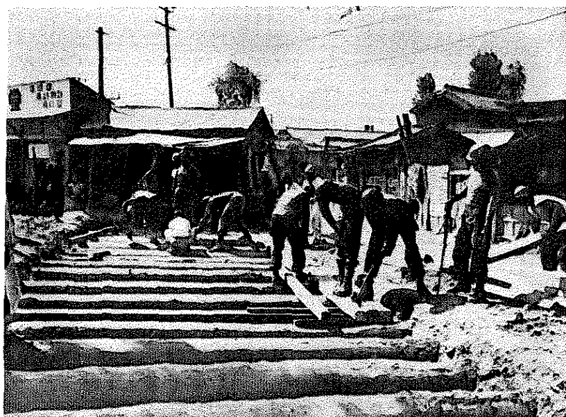
73d Engr (C) Bn bridges a small stream in SCSA, KOREA. (Left)
