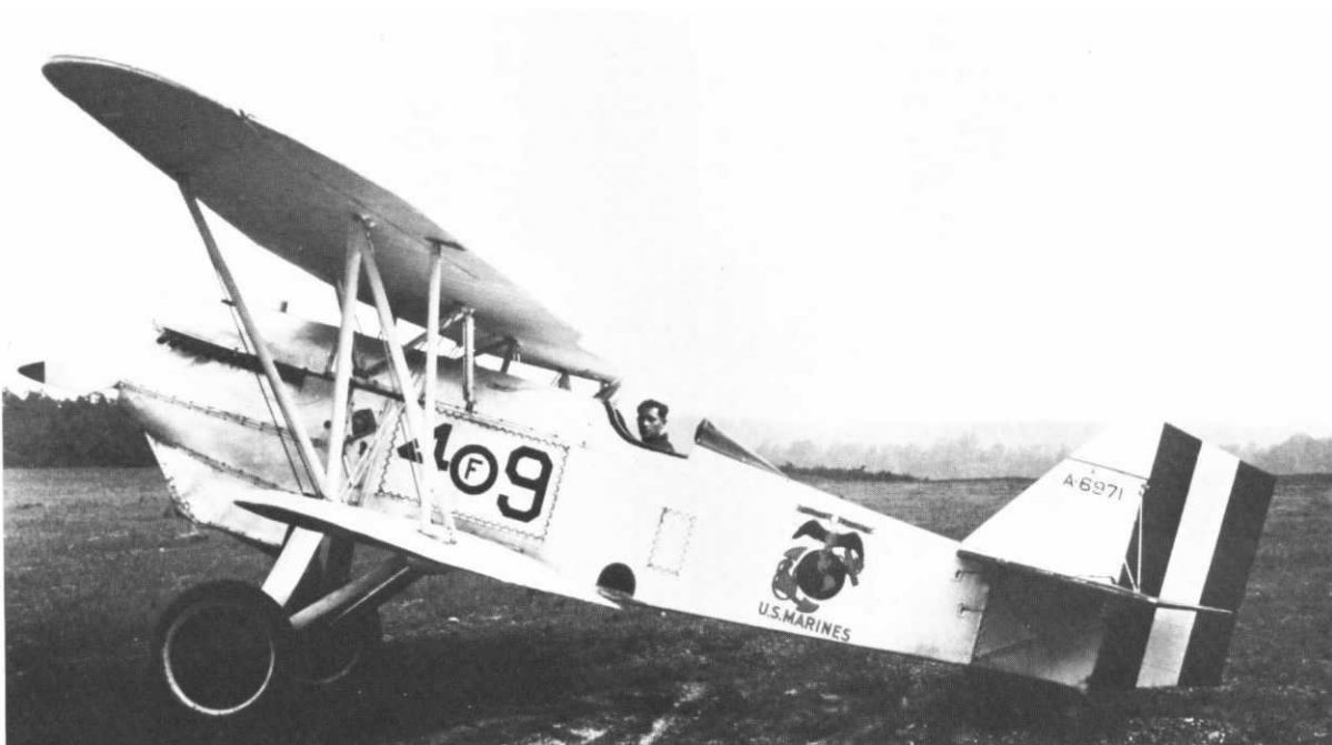
A rare photo of the first model of the Curtiss Hawk fighter, the F6C-1. There were only nine F6C-1s built. (Marine Corps Photo 527944).
