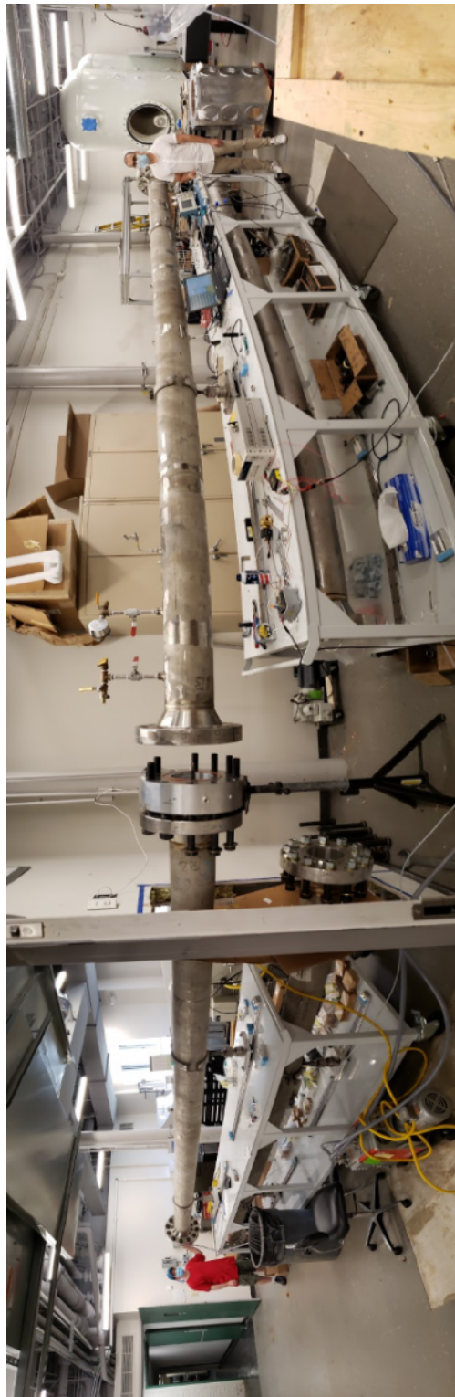
Figure 15: Panorama of the tunnel under construction. Students of Parziales group are pictured: David Shekhtman on left, Ahsan Hameed on right.
