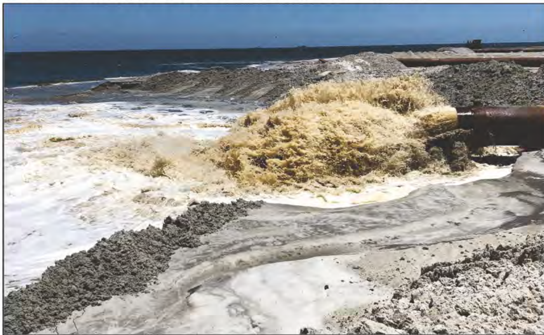
Figure 3-14. Pump-out operations during an active beach nourishment project. Photo courtesy of David Nguyen, ERDC Coastal and Hydraulics Laboratory.
