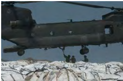
U.S. Army National Guardsmen from Texas attach cargo hooks supporting bags of sand to a CH-47 Chinook helicopter near Lake Pontchartrain in New Orleans, La., on Sept. 10, 2005. The bags are being used to repair a breach, caused by Hurricane Katrina, in the levees around New Orleans. (U.S. Air Force photo by Senior Airman Chris Kerens, 147th Fighter Wing) 050910-F-9177K-056
