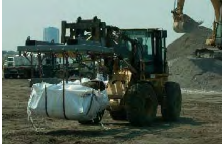
Civilian contractors fill large sandbags used to plug the hole in the levee near Lake Pontchartrain, La., in the aftermath of Hurricane Katrina on Sept. 10, 2005. (U.S. Air Force photo by Senior Airman Chris Kerens, 147th Fighter Wing) 050910-F-9177K-068
