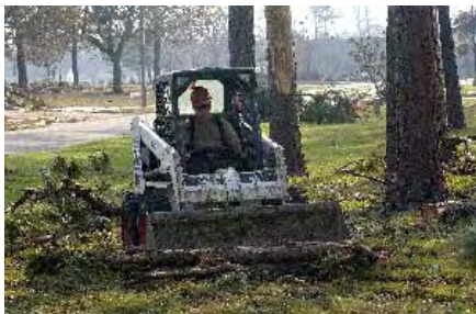
Crews from the 823rd Red Horse Squadron from Hurlburt Field, Fla., were sent to aid in the cleanup effort on Sept. 3, 2005, at Keesler AFB, Miss., after Hurricane Katrina struck the area. (U.S. Air Force photo by Tech. Sgt. Jennifer C. Wallis, 1st Combat Camera Squadron) 050903-F-3820W-203
