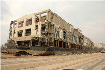
The Grand Casino in Biloxi, Miss., washed ashore to its current resting spot on Sept. 1, 2005, after Hurricane Katrina hit the Gulf Coast. Biloxi was one of the hardest hit areas. (U.S. Air Force photo by Master Sgt. Shaun Withers) 050901-F-1279W-082
