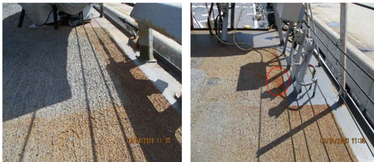
Figure 43 – Close-up of section 3 that received 20% SP10 Grit/80% UPHWJ surface preparation of the deck and power tool cleaning of deck edges and appendages not accessible by UHPWJ
