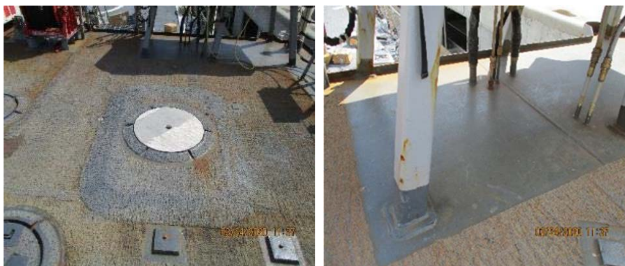
Figure 42 – Close-up of section 2 that received 100% SP6 Grit surface preparation of the deck and appendages
