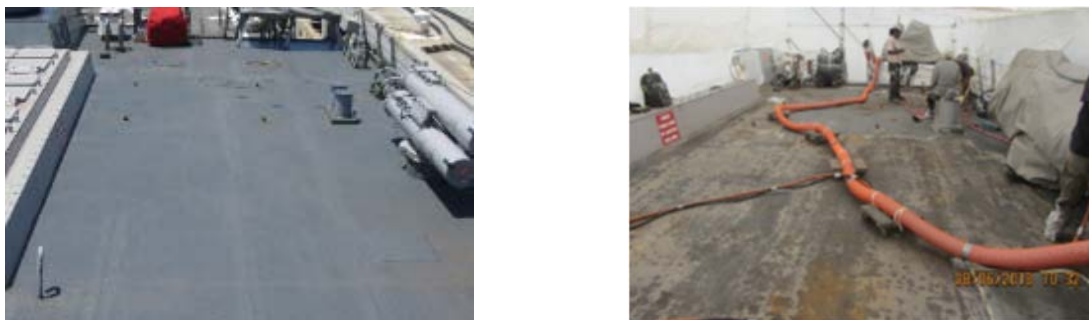
Figure 5 – Initial condition of DDG missile deck (left) and after UHPWJ (right) to remove nonskid coating
