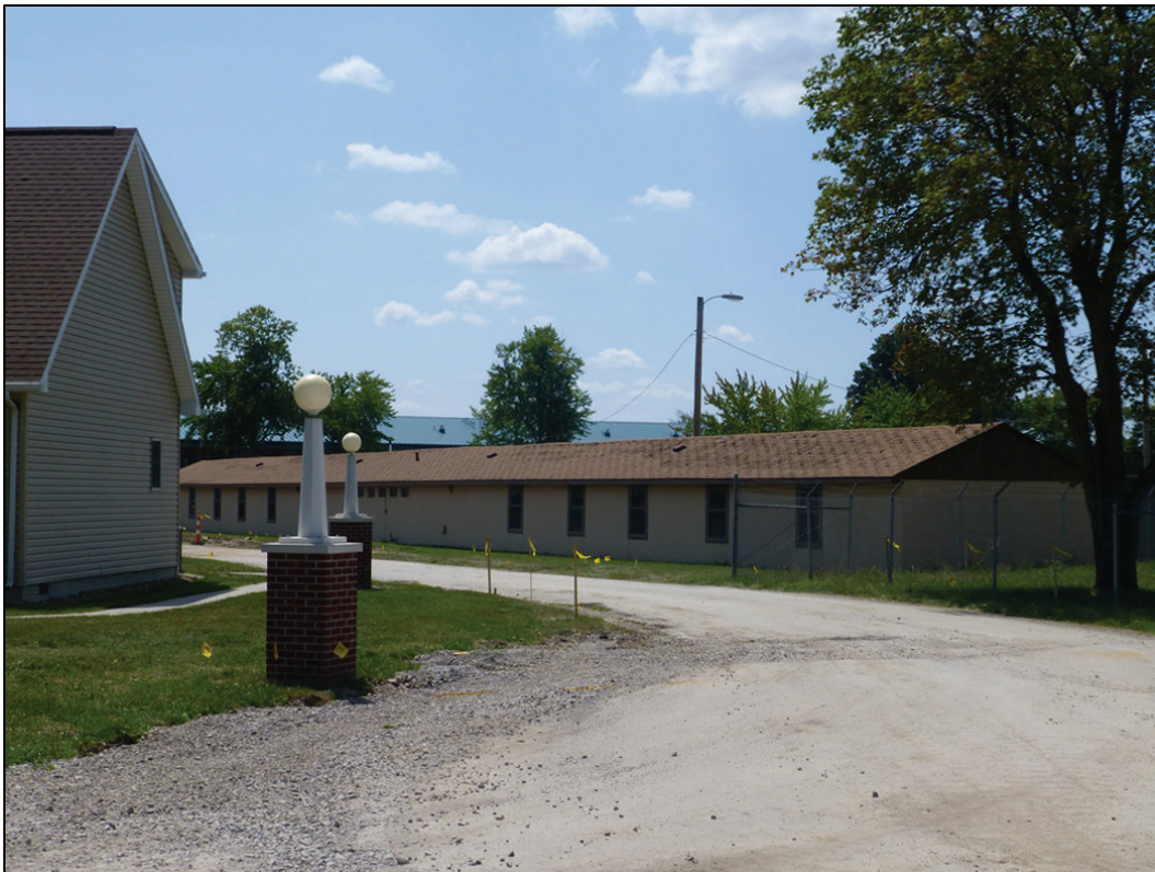
Figure 20. Looking southwest at Building 302 (ERDC-CERL 2017).
