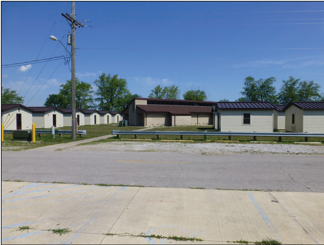
Figure 262. Looking north in Area J towards 1980 latrine/shower building (ERDC-CERL 2017).
