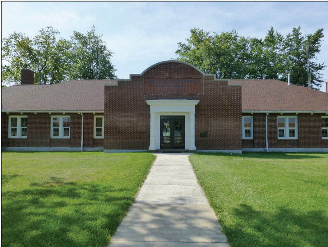
Figure 5. North side of Building 1 (ERDC-CERL 2017).
