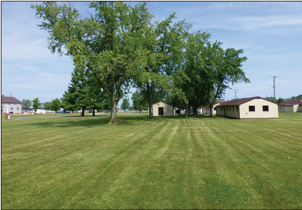
Figure 234. Looking north at WWII administrative buildings in Area G (ERDC-CERL 2017).
