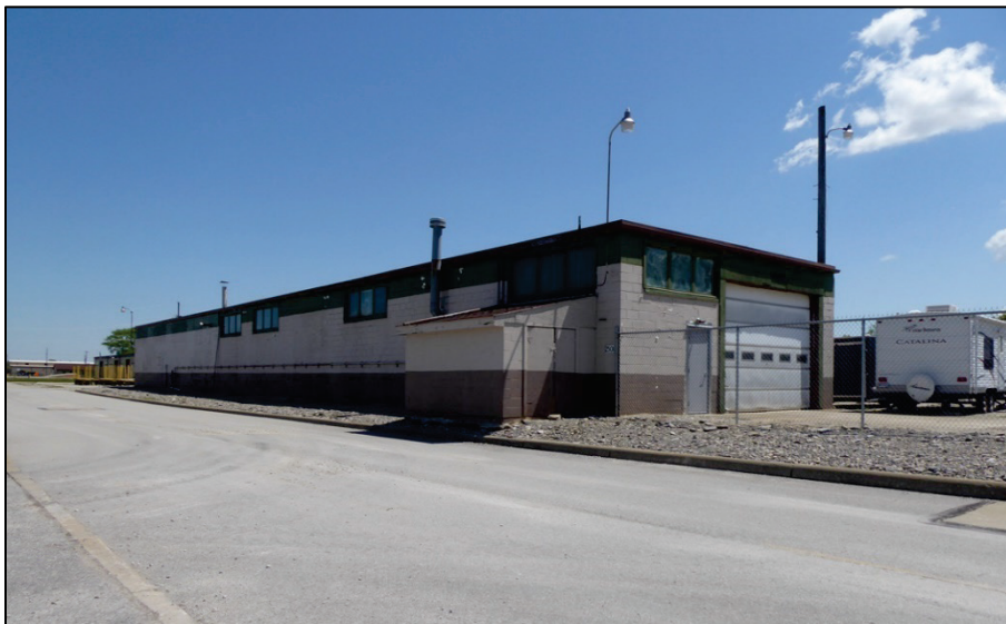
Figure 70. Looking northeast at Building 2501 (ERDC-CERL 2017).
