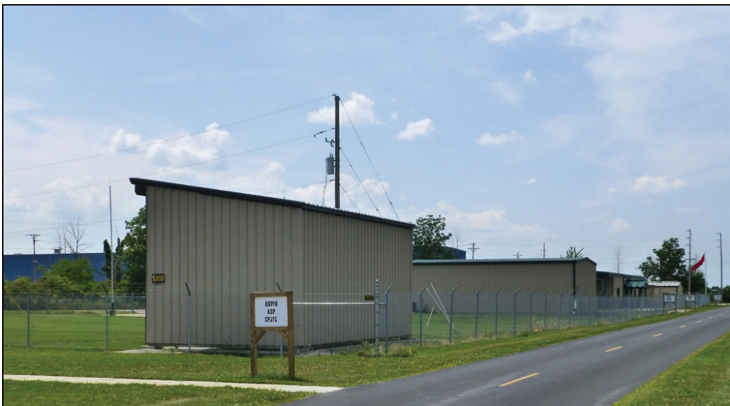
Figure 104. Looking southwest at Building 5204 (ERDC-CERL 2017).
