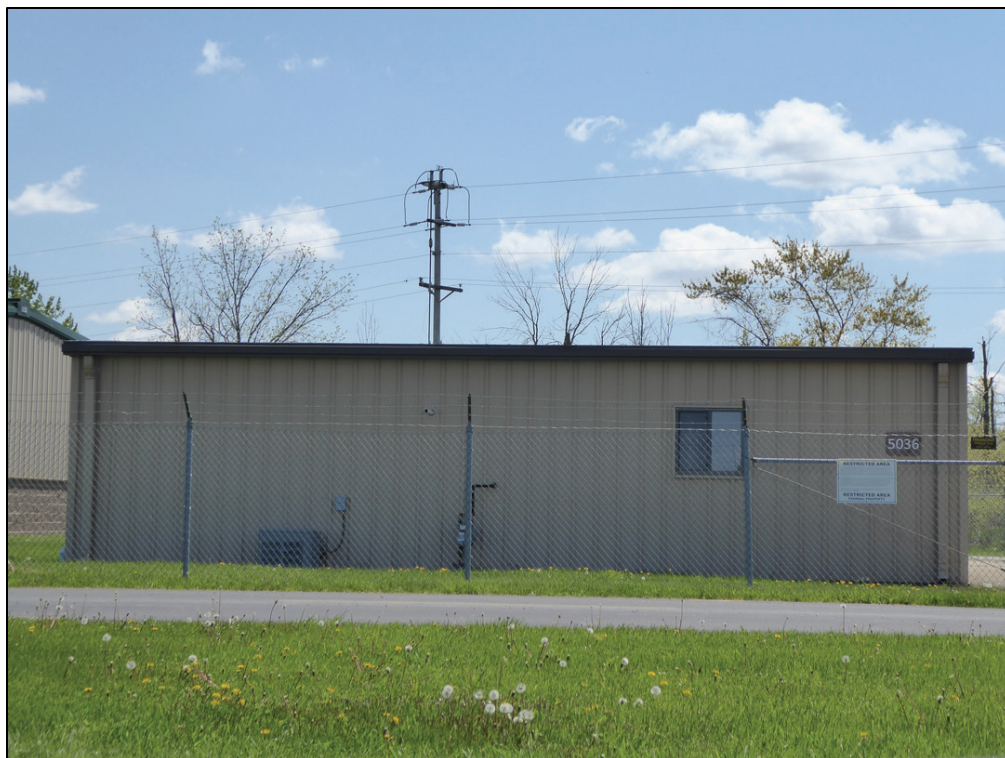
Figure 97. North facade of Building 5036 (ERDC-CERL 2019).
