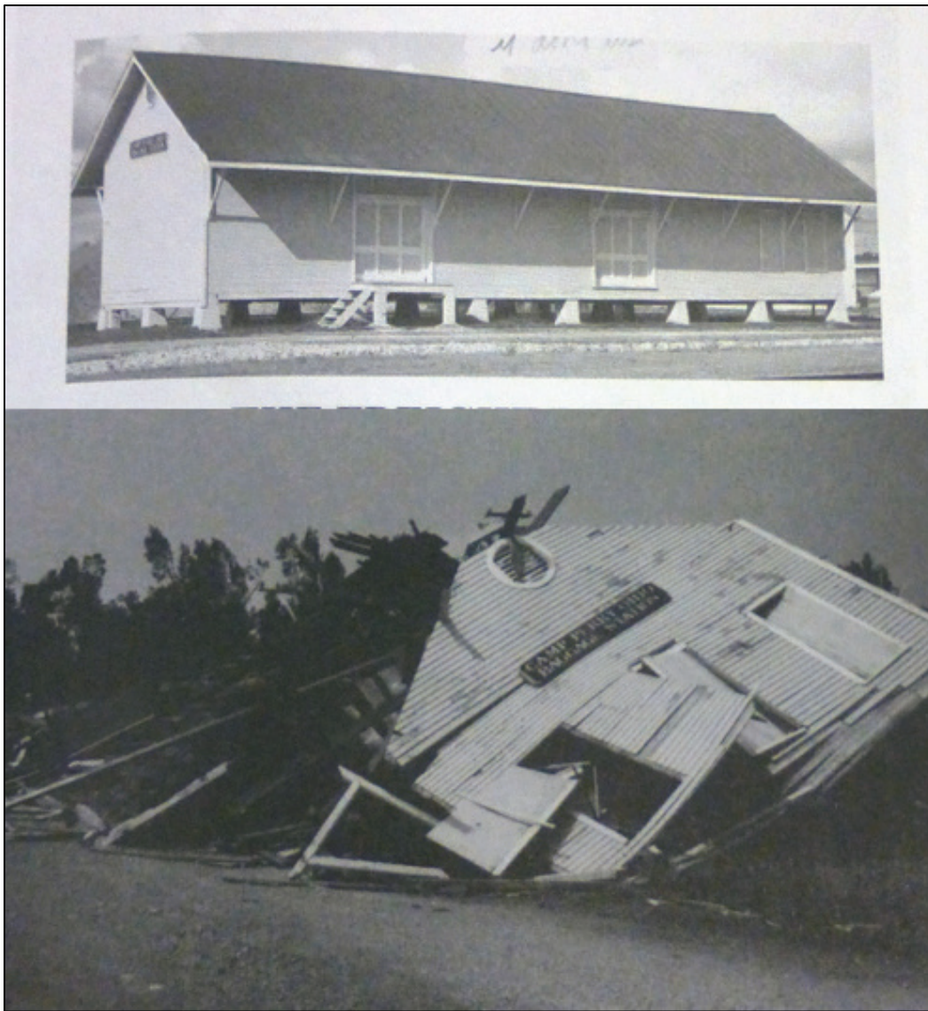
Figure 281. Images of former freight depot, which was destroyed by tornado in 1998 (Camp Perry).
