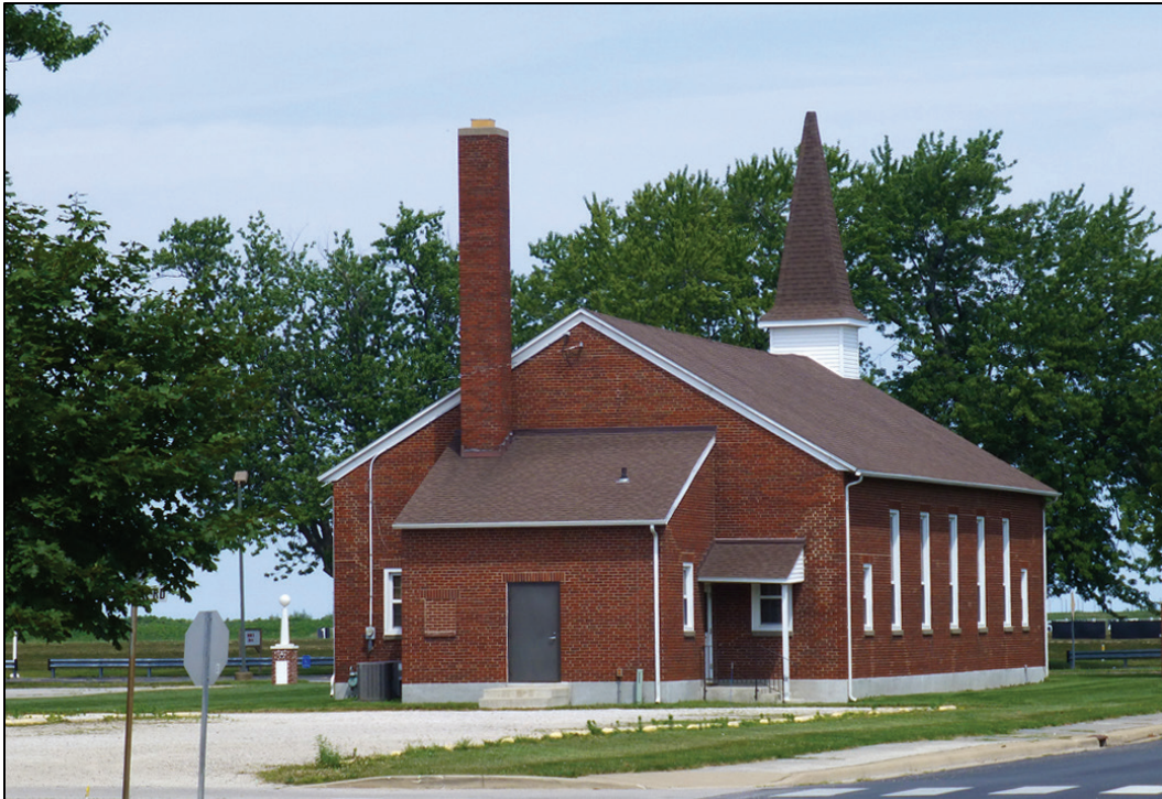
Figure 44. Looking north at Building 1003 (ERDC-CERL 2017).
