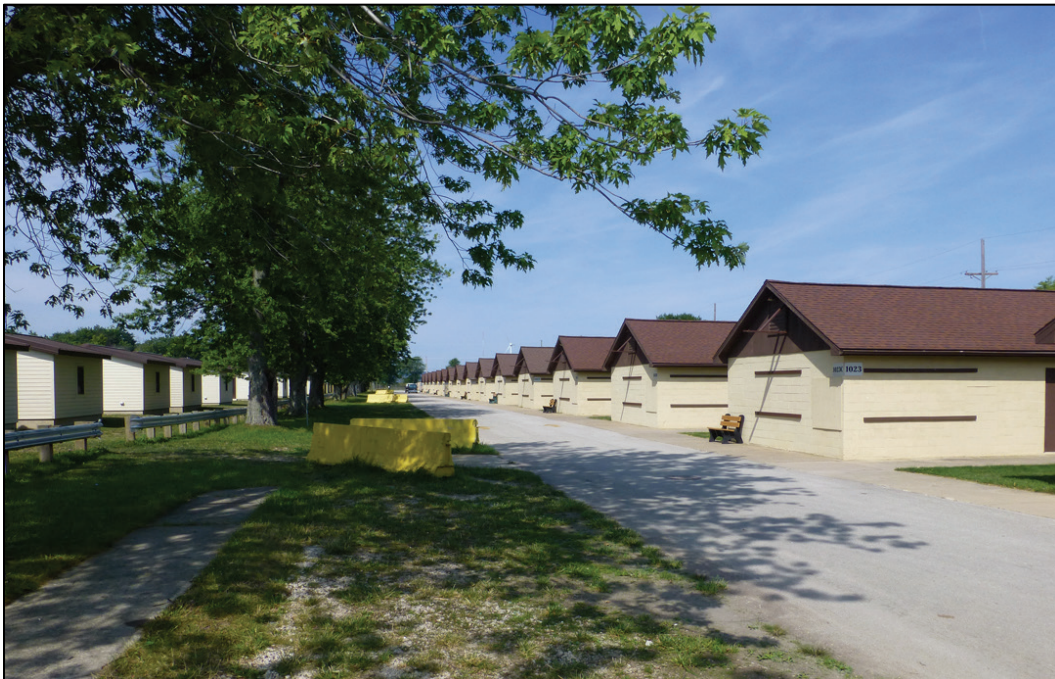
Figure 253. Looking west along Donahey Road with the WWII mess halls on the right in Area I (ERDC-CERL 2017).
