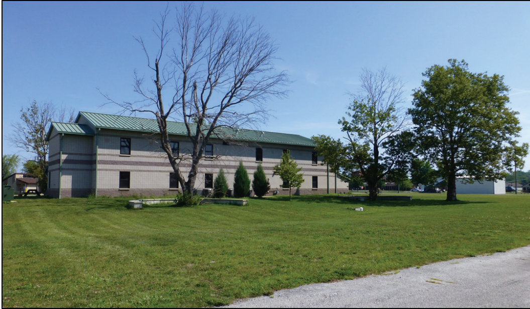
Figure 48. Looking north at Building 1750 (ERDC-CERL 2017).
