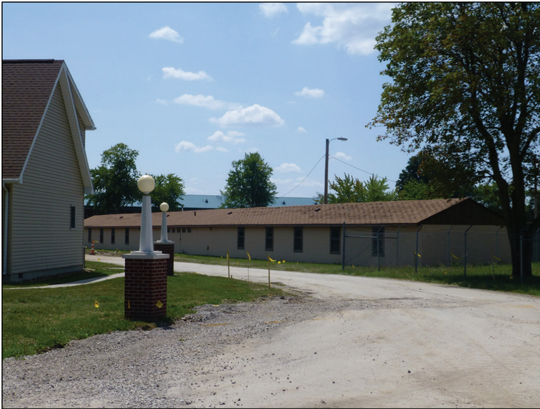
Figure 212. View south along Critchfield Road towards Building 302 (ERDC-CERL 2017).
