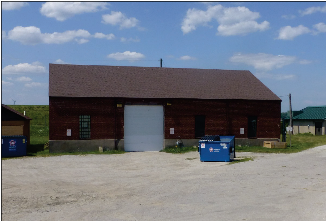
Figure 23. Looking west at Building 403 (center) with Building 402 slightly visible on left and Building 402 slightly visible to right (ERDC-CERL 2017).
