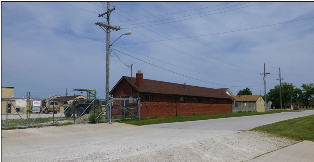
Figure 64. Looking northeast at Building 2023 (ERDC-CERL 2017).
