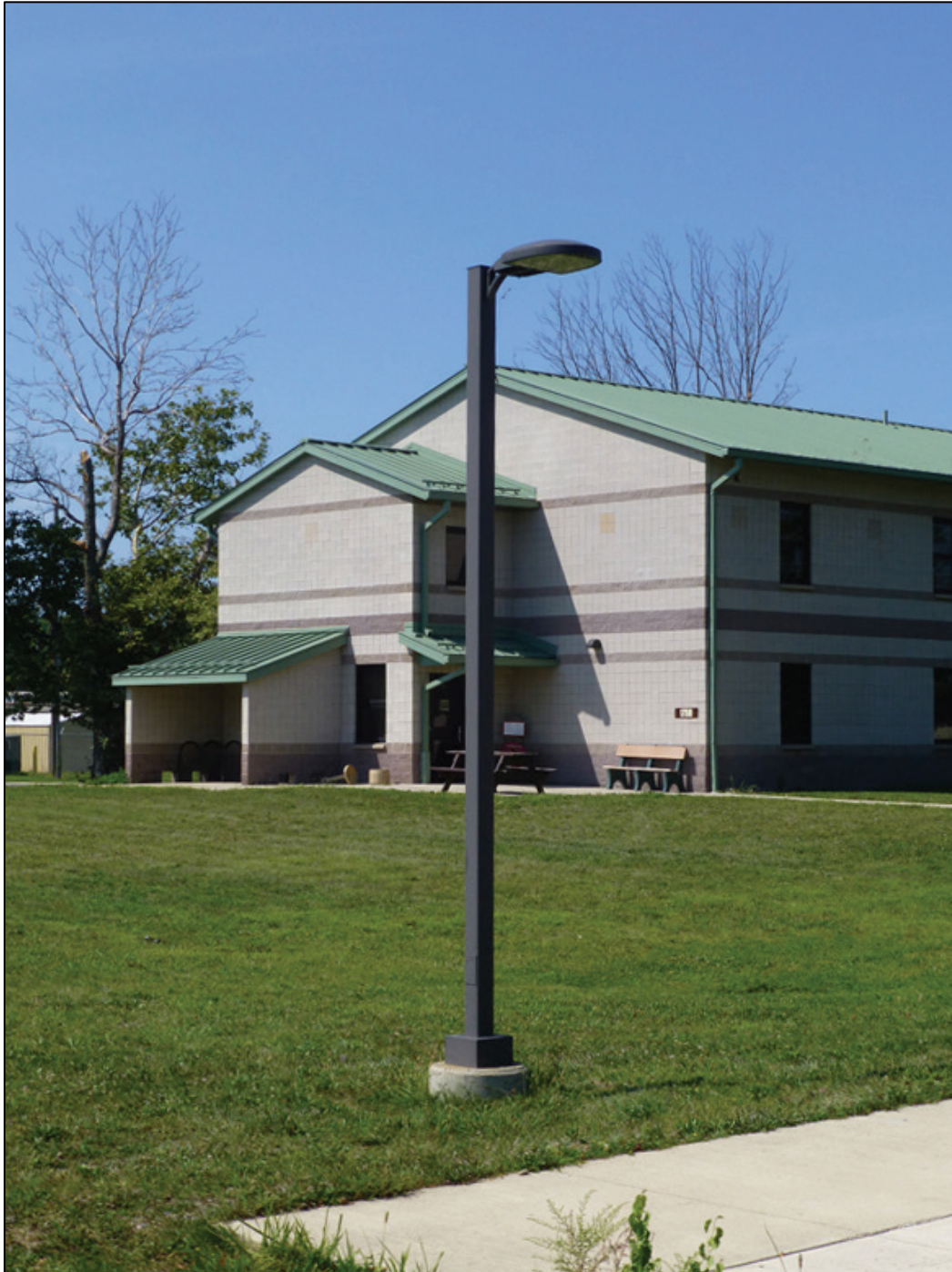
Figure 47. Looking southwest at Building 1750 (ERDC-CERL 2017).
