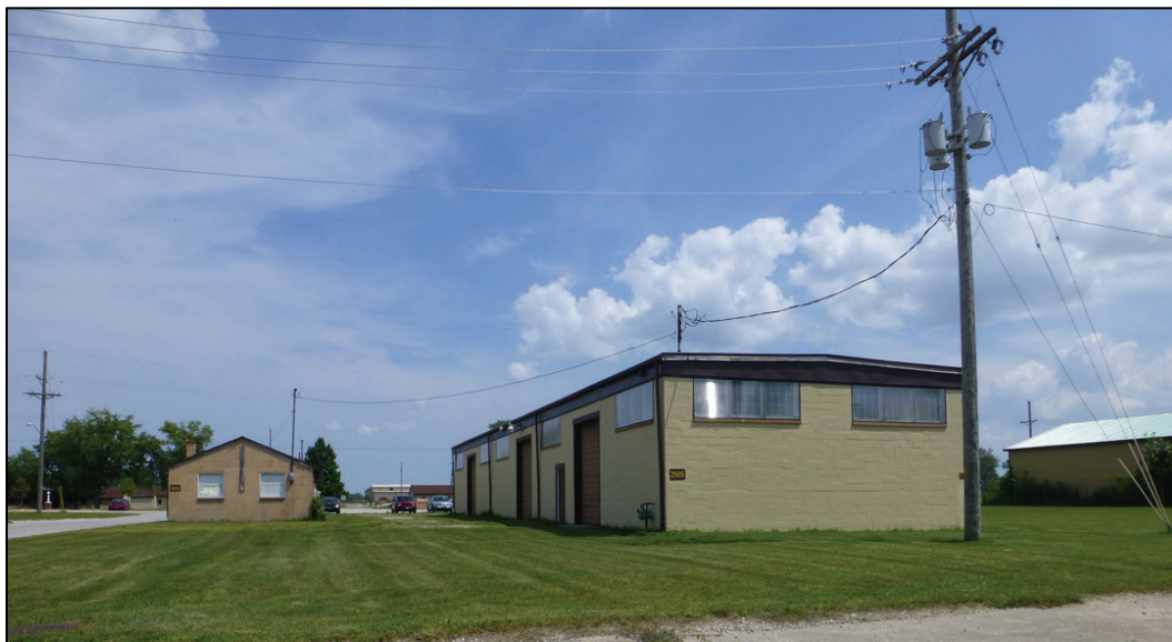
Figure 71. Looking east with Building 2404 (left) and Building 2505 (right) (ERDC-CERL 2017).
