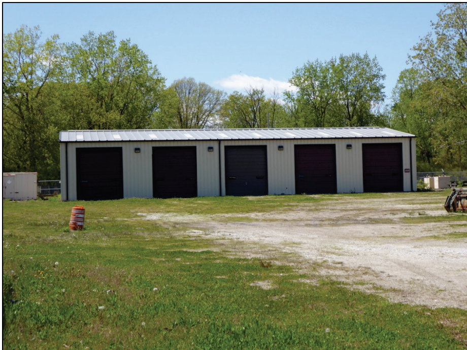
Figure 66. East facade of Building 2026 (ERDC-CERL 2019).
