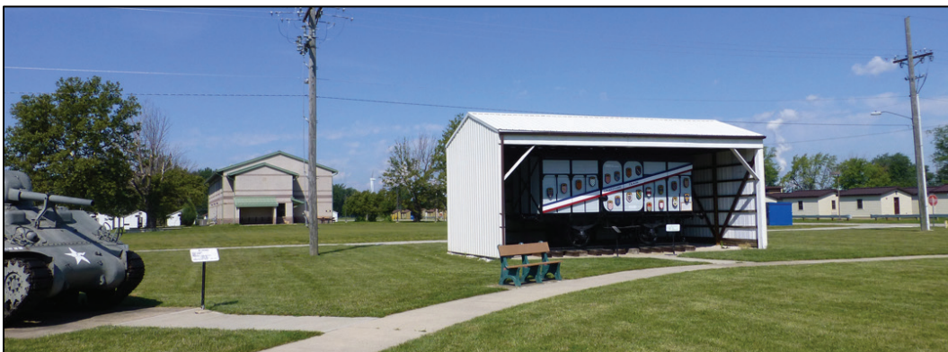
Figure 49. Looking west at Gratitude Train monument (Building 1751) and canopy (Building 1749) (ERDC-CERL 2017).
