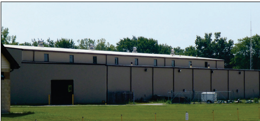
Figure 76. Looking southeast at Building 2807 (ERDC-CERL 2017).
