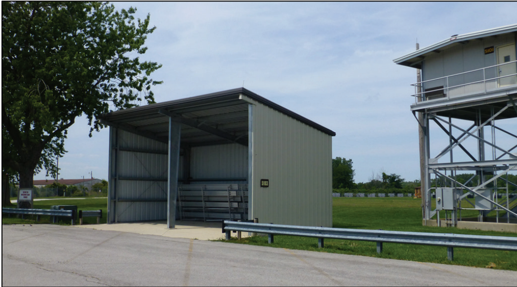
Figure 102. Looking northeast at Building 5103 (ERDC-CERL 2017).
