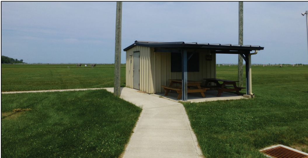
Figure 101. Looking north with Building 5102 (ERDC-CERL 2017).
