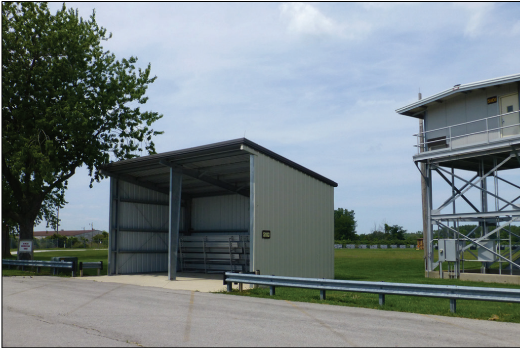
Figure 293. Looking north at Building 5103 at the western end of Area 0 (ERDC-CERL 2017).
