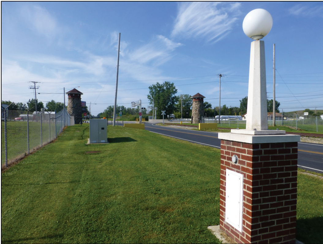
Figure 117. Reconstructed street lamp post on Niagara Road near the Main Gate (ERDC-CERL 2017).
