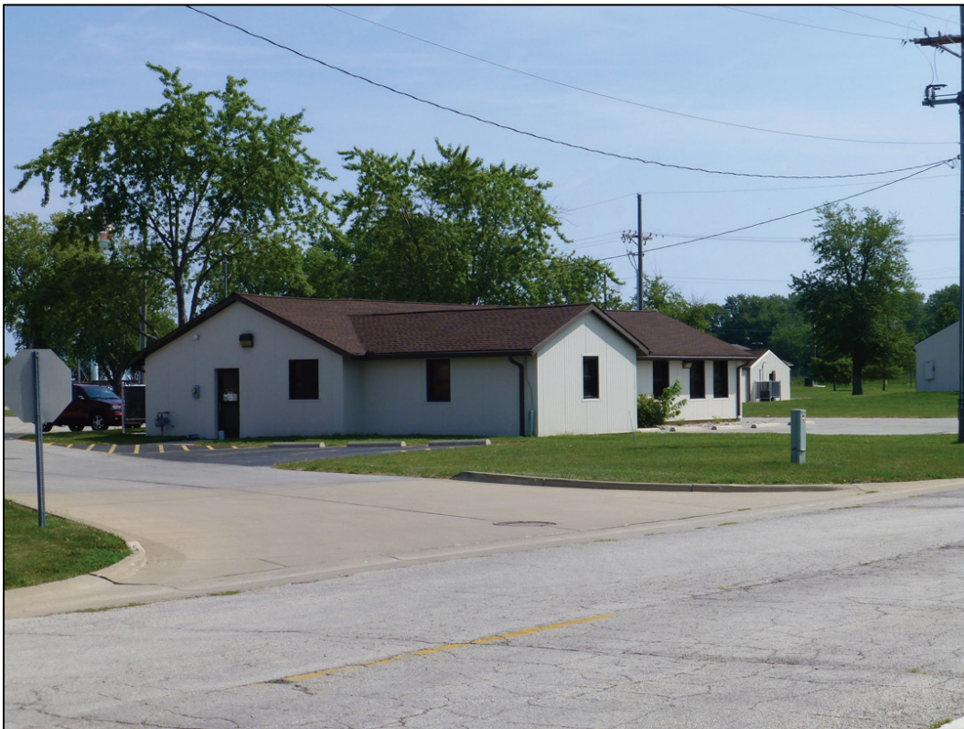
Figure 15. Looking northeast at Building 8 (ERDC-CERL 2017).
