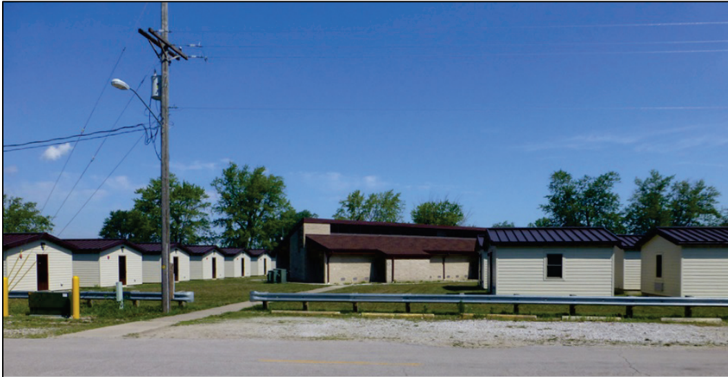
Figure 113. Looking north at latrine (Building EF), in center (ERDC-CERL 2017).
