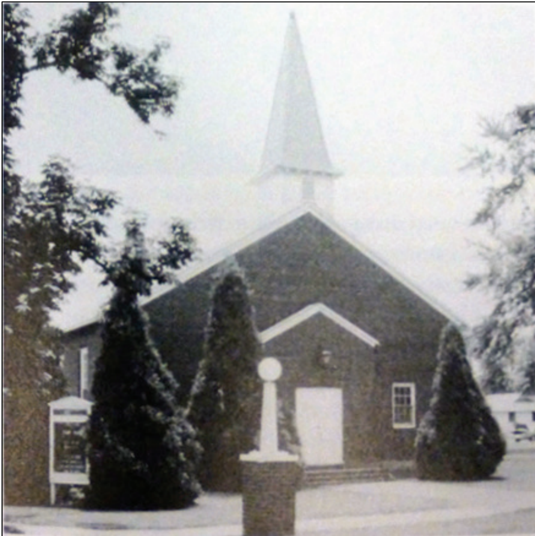
Figure 247. Historic photograph of chapel (Building 1003), date unknown (Camp Perry).
