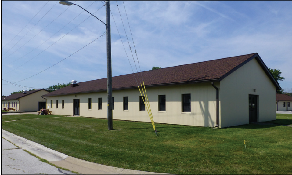
Figure 51. Looking southwest at Building 1804 (ERDC-CERL 2017).
