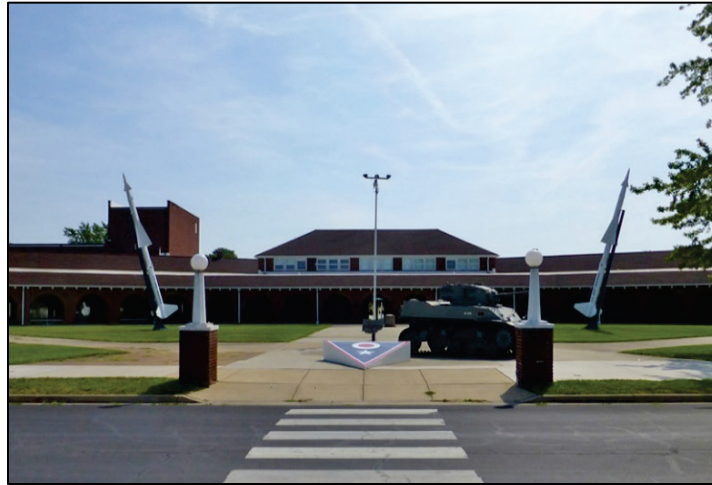
Figure 130. View looking east toward Building 3, with missiles and tank memorials (ERDC-CERL 2017).
