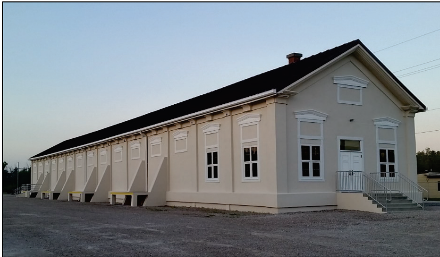
Figure 60. Looking west at Building 2009 (Camp Perry 2017).
