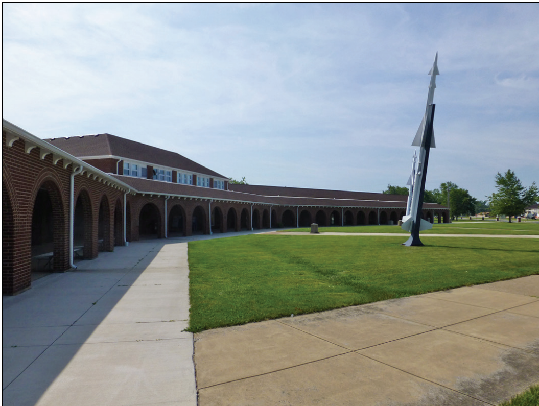
Figure 9. Looking southeast at Building 3 (ERDC-CERL 2017).
