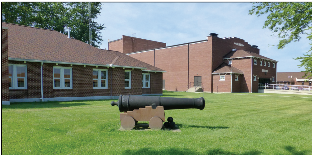
Figure 222. Looking southwest in Area F, with Building 1 on the left and Building 2 on the right (ERDC-CERL 2017).
