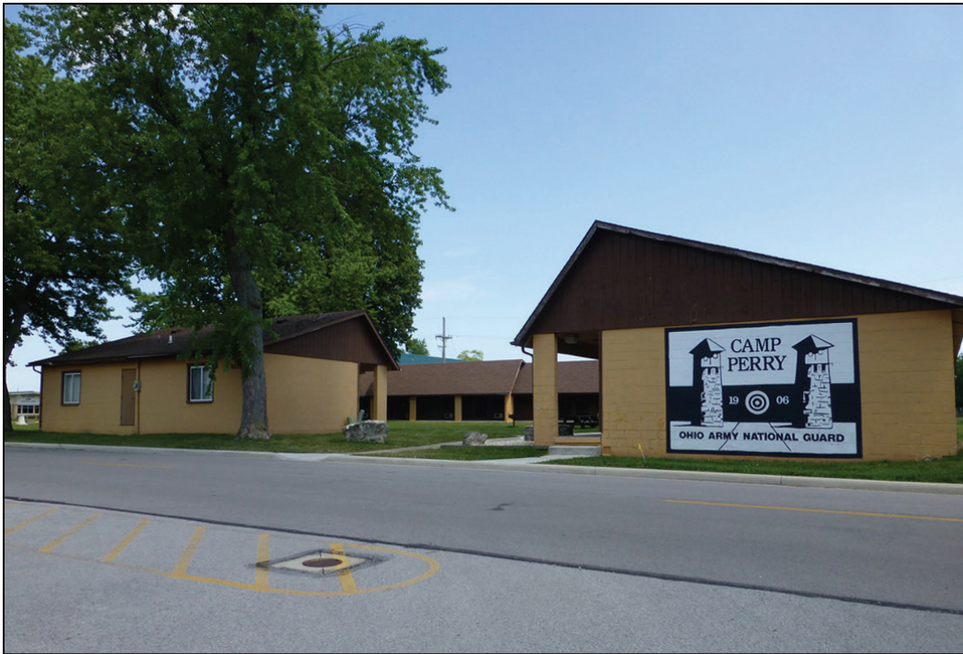
Figure 16. Looking east at Building 120 and Building 150, with Building 160 in background, center (ERDC-CERL 2017).
