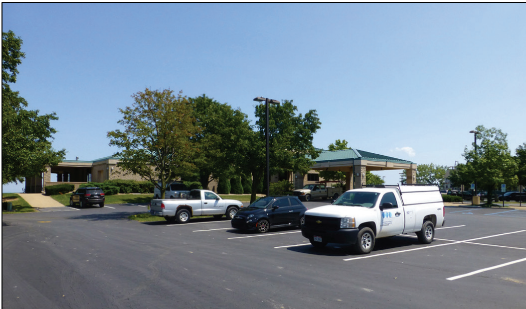
Figure 32. Looking north at Building 600 (ERDC-CERL 2017).
