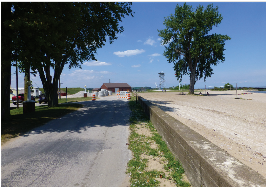
Figure 209. Looking west along Critchfield Road at the retaining wall and the beach towards the ice house (Building 402) in Area E (ERDC-CERL 2017).
