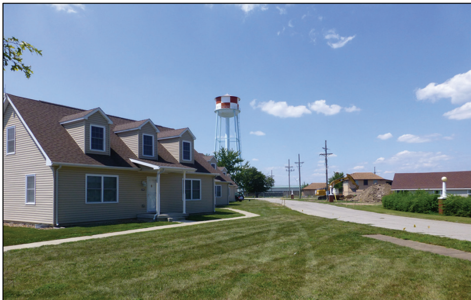
Figure 30. Looking southwest at Building 522, shown at left (ERDC-CERL 2017).
