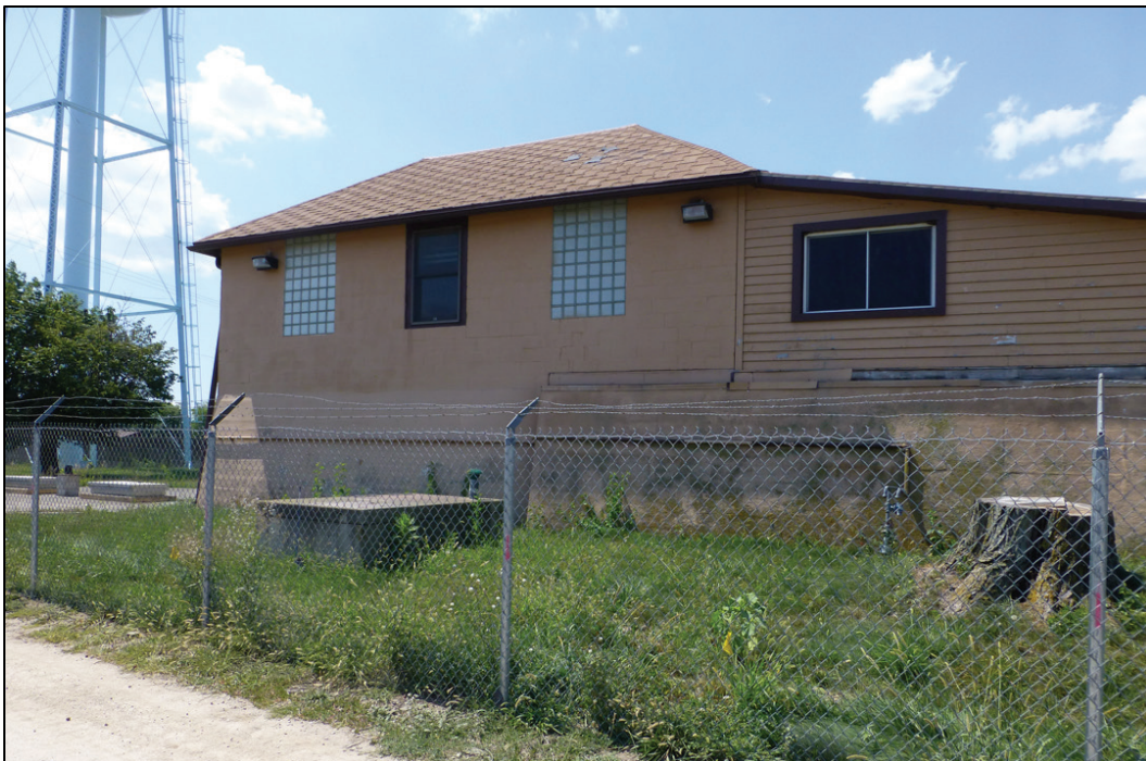
Figure 25. Looking southwest at Building 492 (ERDC-CERL 2017).
