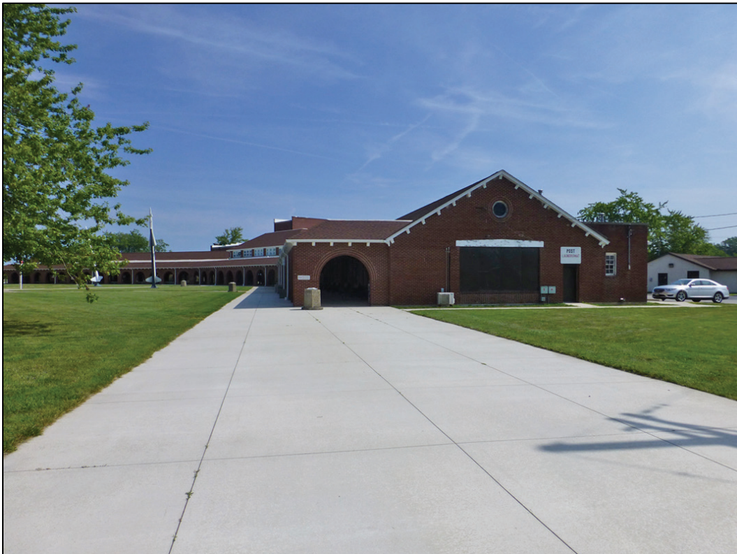
Figure 11. Looking north at Building 3 (ERDC-CERL 2017).
