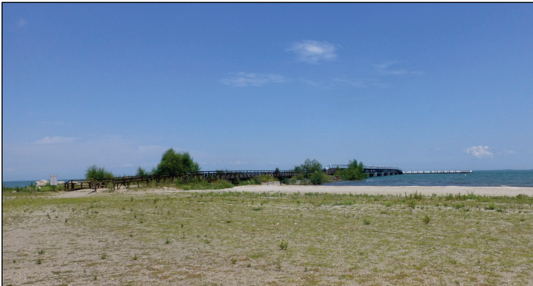
Figure 211. View of pier, bridge, and breakwater (ERDC-CERL 2017).
