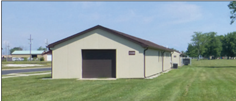
Figure 87. Looking north at Building 3100 (ERDC-CERL 2017).
