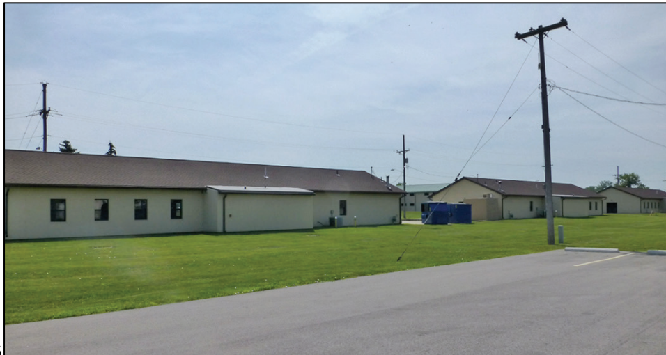
Figure 52. Looking southeast at Building 1804 (left) and Building 1845 (right) (ERDC-CERL 2017).
