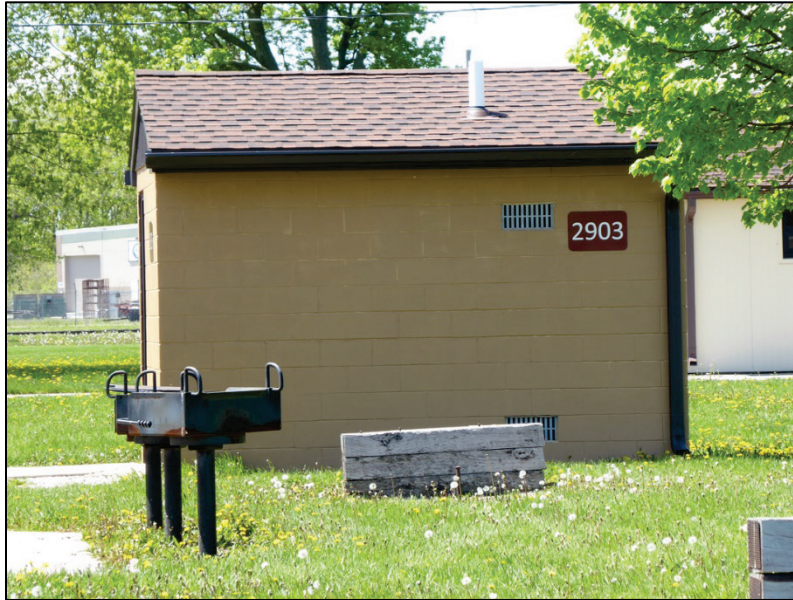
Figure 85. South facade of Building 2903 (ERDC-CERL 2019).
