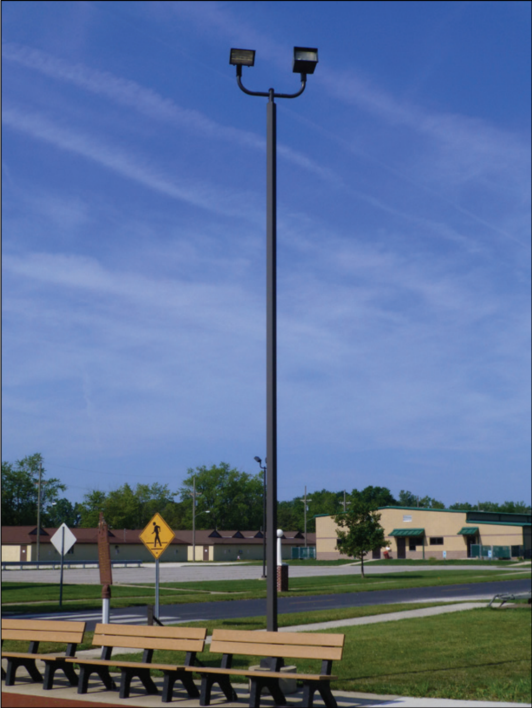
Figure 147. Lighting in Shooter Memorial Plaza (ERDC-CERL 2017).
