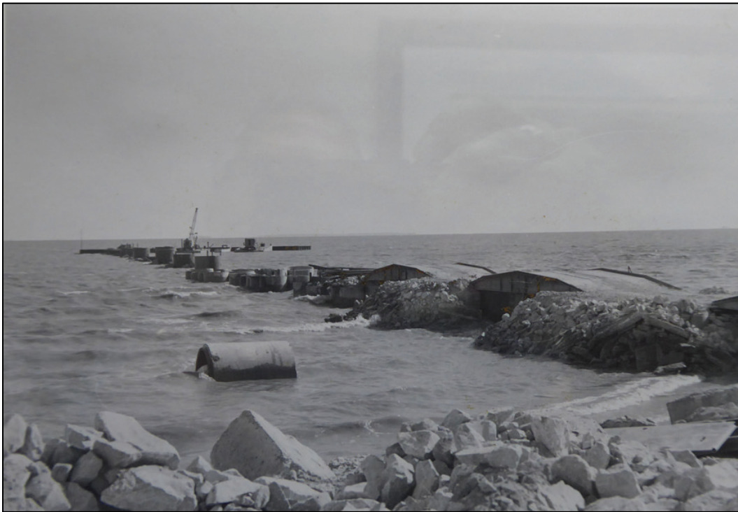
Figure 204. Photo showing reconstruction of pier in 1975 (Camp Perry).
