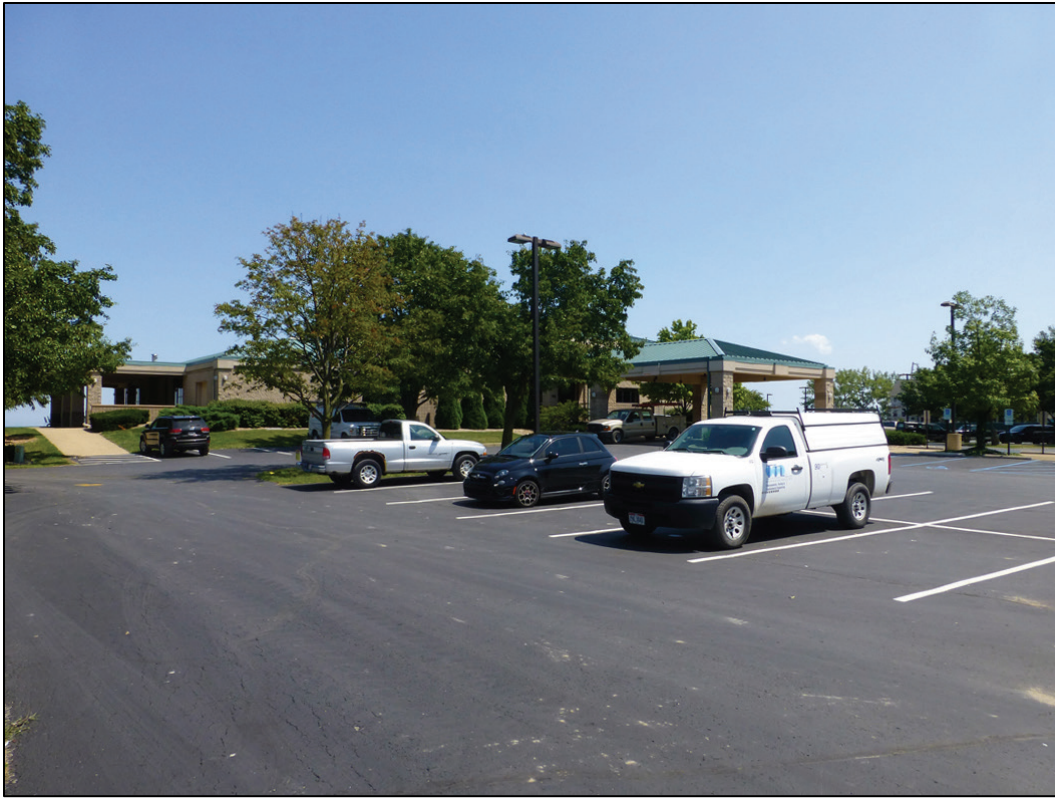
Figure 206. Looking north towards Building 600 in Area E (ERDC-CERL 2017).
