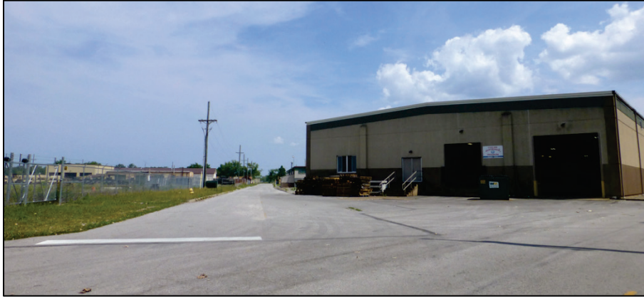
Figure 69. Looking southeast at Building 2500 (ERDC-CERL 2017).
