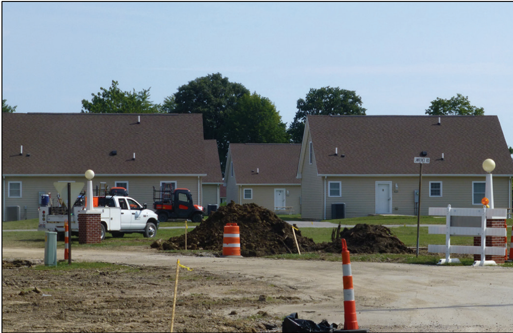
Figure 31. Looking northeast at the rear of 524 and 525 (ERDC-CERL 2017).
