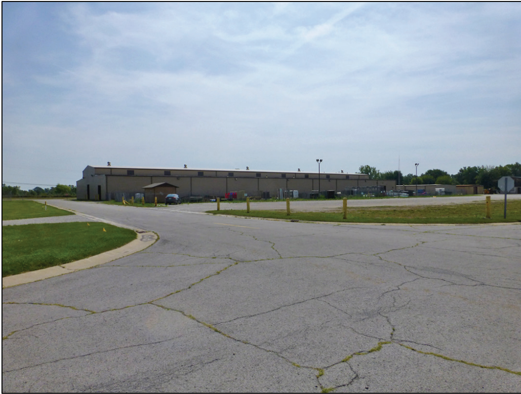
Figure 183. Looking southeast over Area C (ERDC-CERL 2017).
