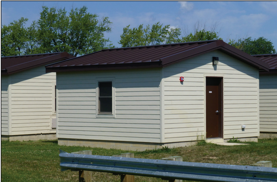
Figure 110. Looking northwest at hutments (ERDC-CERL 2017).
