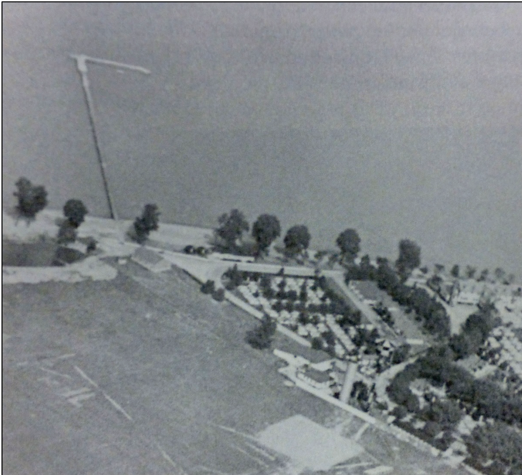
Figure 202. Aerial of new pier and breakwater, 1934 (Camp Perry).
