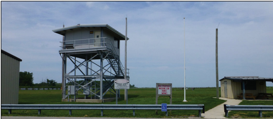
Figure 106. Looking north at Building T5101 on the left (ERDC-CERL 2017).
