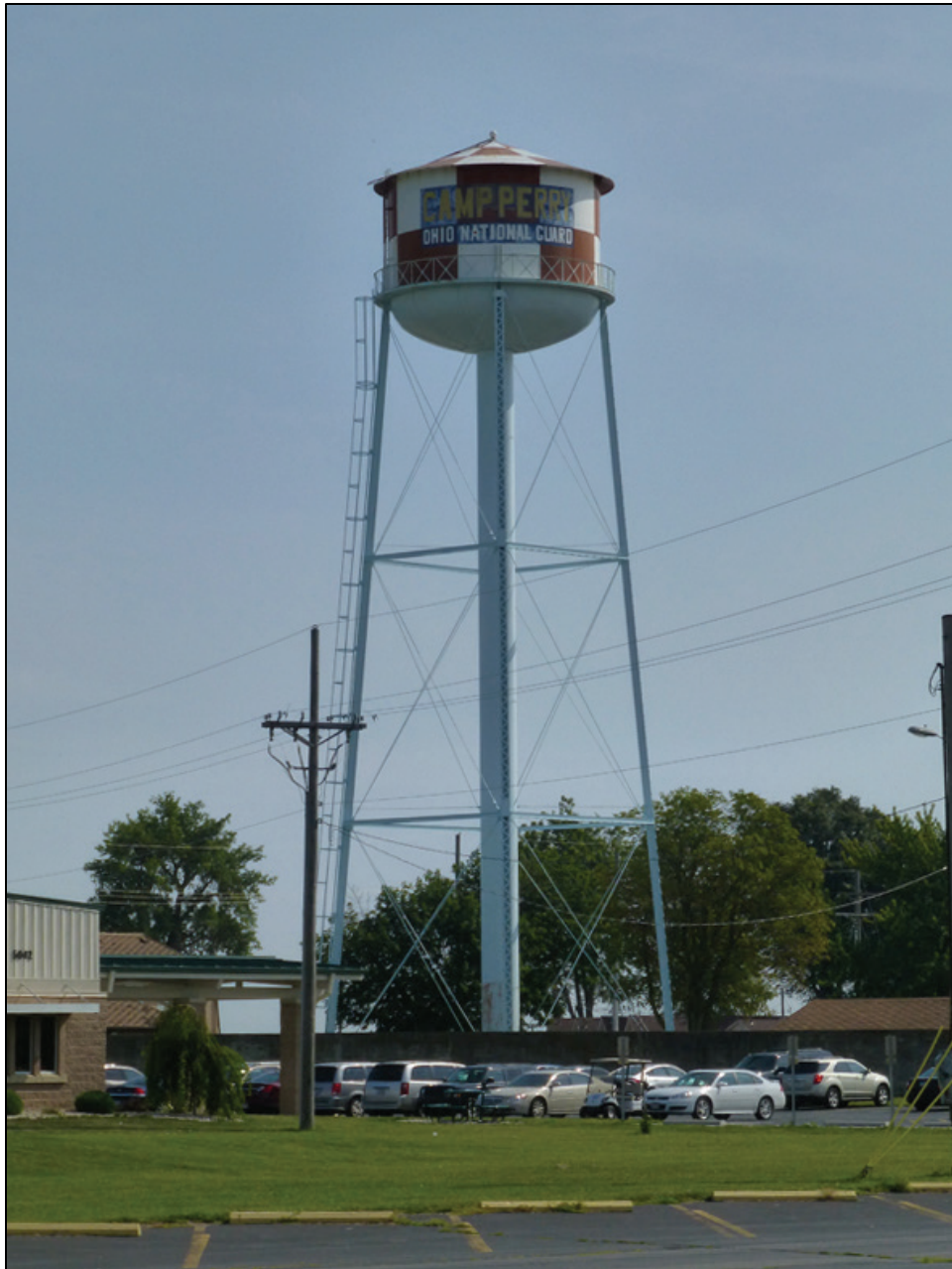
Figure 19. Looking north at Building 301 (ERDC-CERL 2017).
