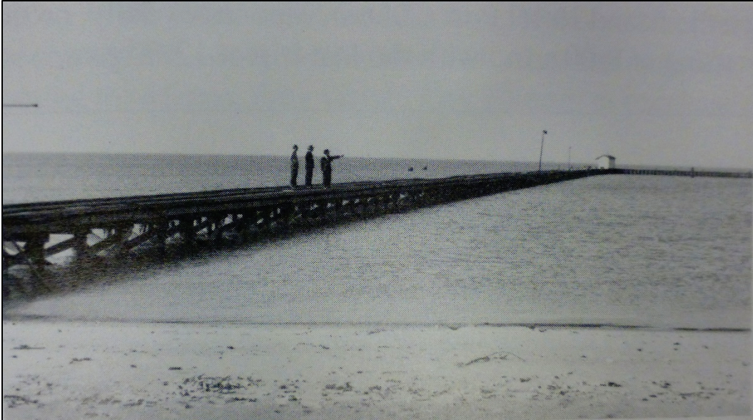
Figure 201. Photograph of pier that was added in 1934, date unknown (Camp Perry).
