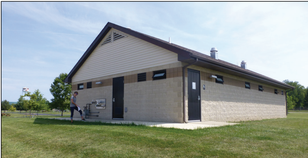
Figure 68. Southwest oblique of Building 2201, which is a latrine for the camping area (ERDC-CERL 2017).
