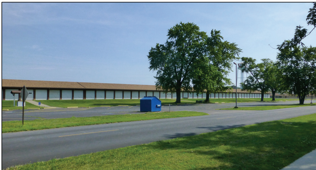
Figure 99. Looking north at Building 5039 (ERDC-CERL 2017).
