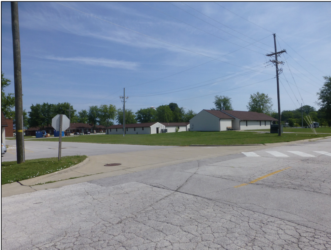
Figure 224. Looking northeast into Area F (ERDC-CERL 2017).
