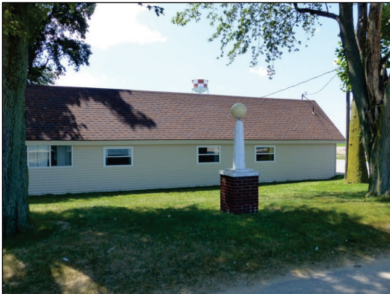
Figure 28. Looking south at 501 (ERDC-CERL 2017).
