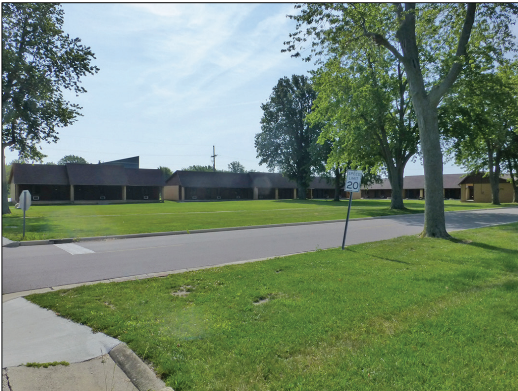
Figure 17. Looking east at 100, 120, 150, 160, and 170 (ERDC-CERL 2017).
