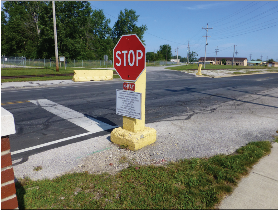
Figure 142. Stop sign on concrete structure (ERDC-CERL 2017).
