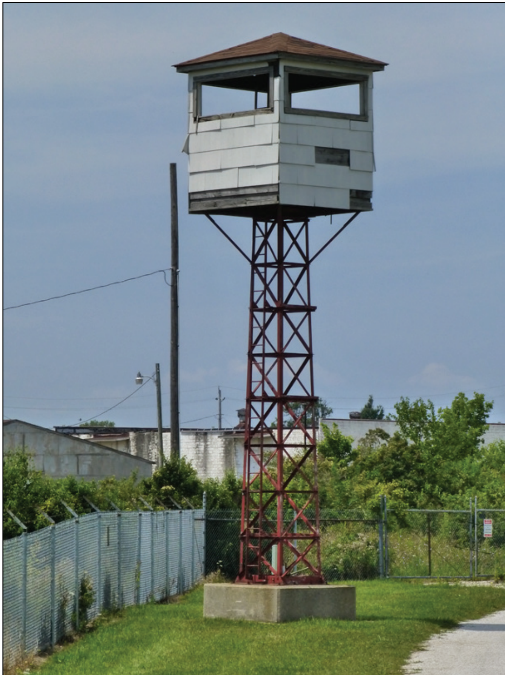
Figure 94. Looking northwest at Building 5002 (ERDC-CERL 2017).
