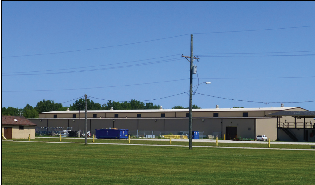
Figure 77. West side of Building 2807 (ERDC-CERL 2017).
