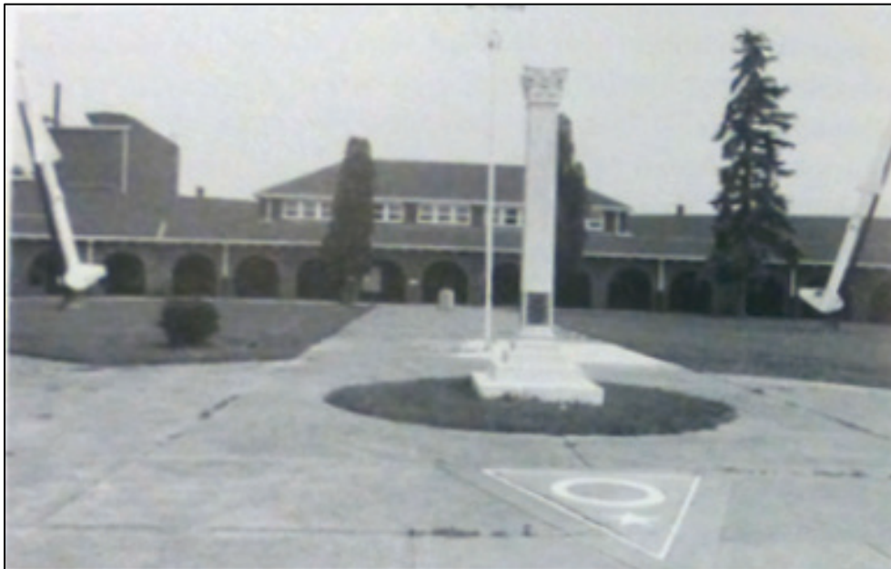
Figure 238. The Critchfield Monument's original location in front of Building 3, ca. 1987 (Camp Perry).
