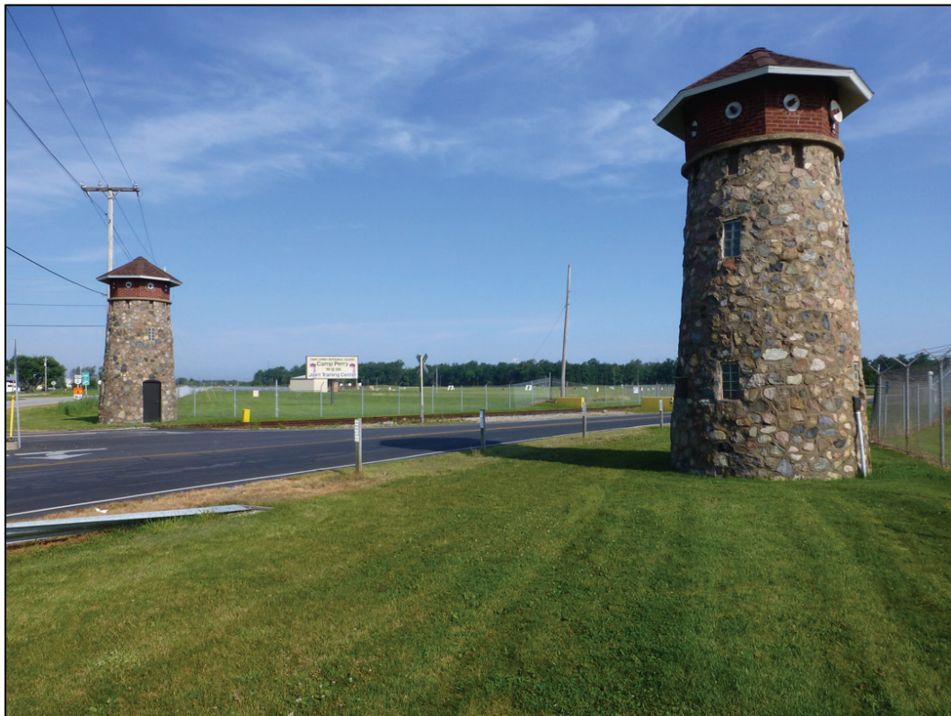
Figure 154. Looking northwest at Main Gate (ERDC-CERL 2017).
