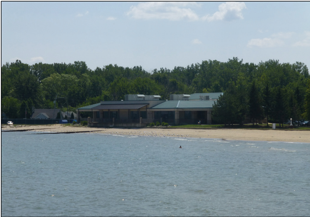
Figure 33. Looking southeast at Building 600 with Lake Erie in foreground (ERDC-CERL 2017).
