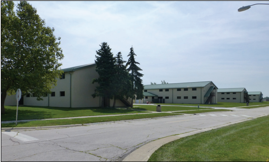
Figure 53. Looking southeast toward Buildings 1805, 1846, 2146, and 2305 (ERDC-CERL 2017).
