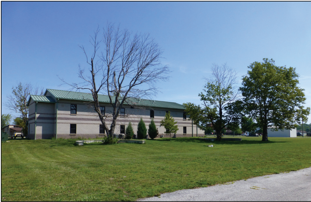
Figure 270. Looking north in Area K towards the barracks (Building 1750) (ERDC-CERL 2017).
