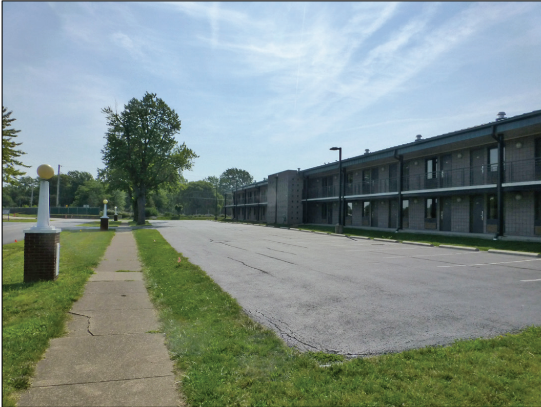
Figure 18. Looking southeast at Building 200 (ERDC-CERL 2017).
