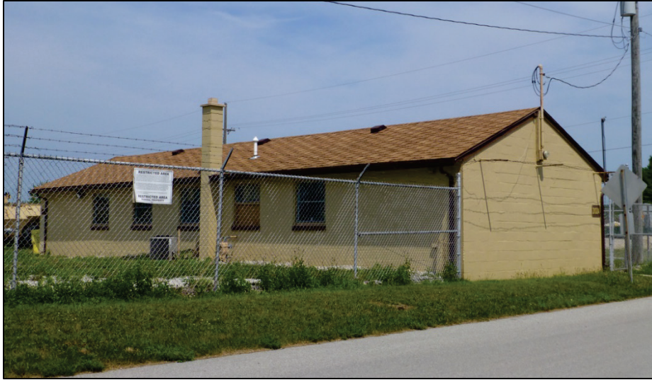
Figure 65. Looking northeast at Building 2024 (ERDC-CERL 2017).
