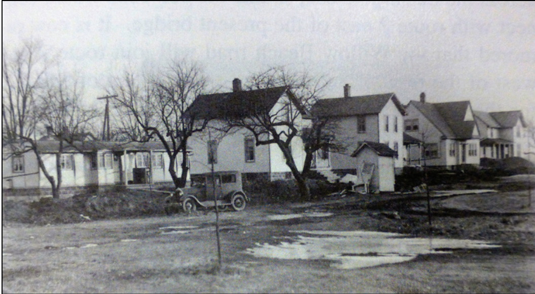
Figure 181. Relocated Buildings 3207, 3208 and 3209, ca. 1938 (Camp Perry).
