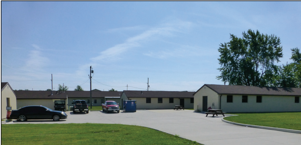
Figure 67. Looking east at Building 2142 on the right with Building 2143 behind (ERDC-CERL 2017).
