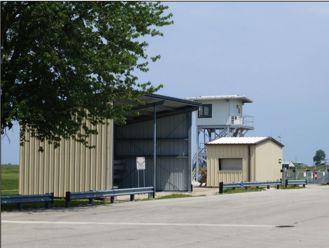
Figure 294. Looking northeast at Building 5203 and 5202 in Area 0 (ERDC-CERL 2017).
