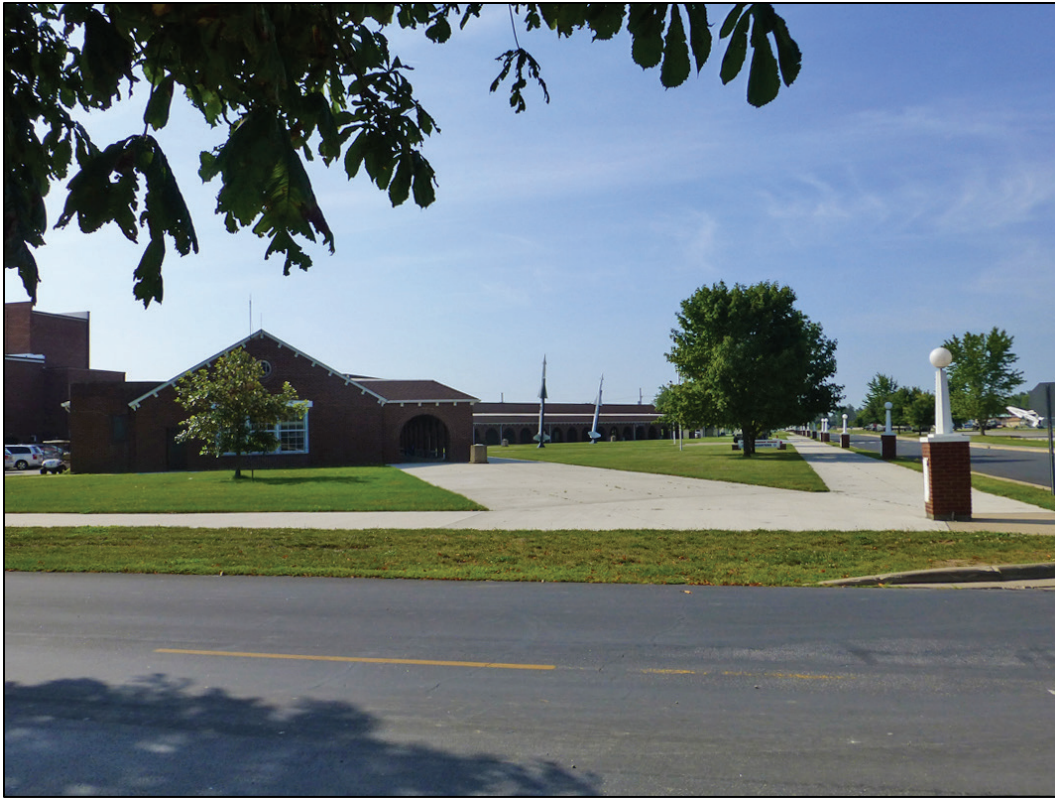
Figure 223. Looking south at Building 3 in Area F (ERDC-CERL 2017).
