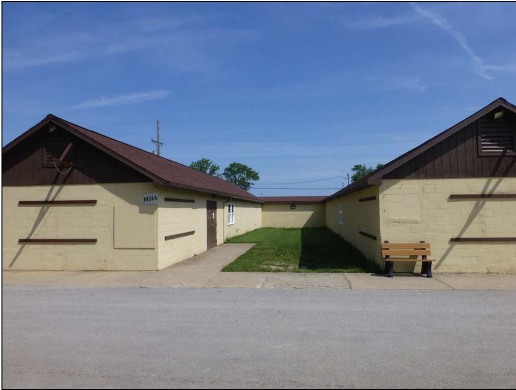
Figure 39. Looking north at Building 1024 (ERDC-CERL 2017).
