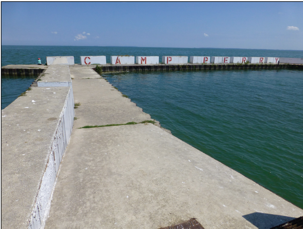
Figure 112. Looking north at breakwater (ERDC-CERL 2017).
