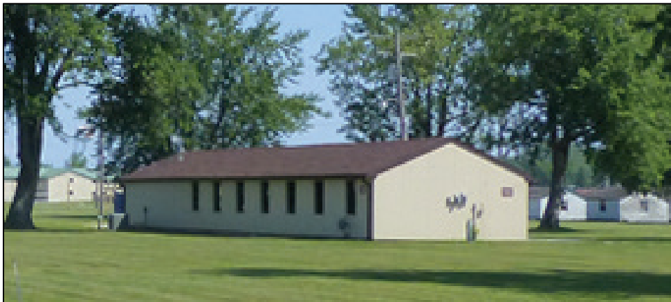
Figure 88. Looking north towards Building 3082 (ERDC-CERL 2017).
