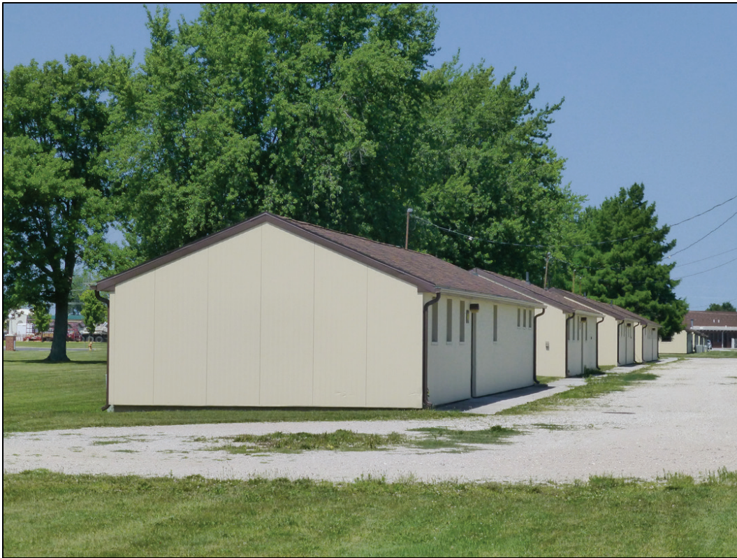
Figure 75. Looking northwest towards 2746, 2702, 2648, and 2603 (ERDC-CERL 2017).
