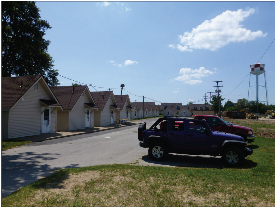
Figure 29. Looking south at rear of Buildings 501, 502, 503 and 504, on left (ERDC-CERL 2017).
