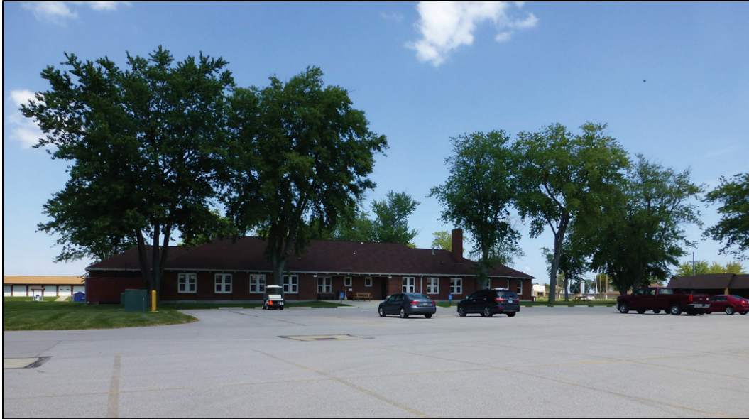
Figure 6. South side of Building 1 (ERDC-CERL 2017).
