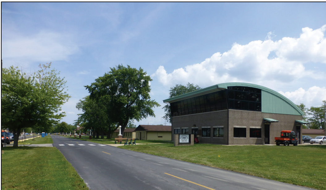
Figure 40. Looking west with Building 930 on the right (ERDC-CERL 2017).
