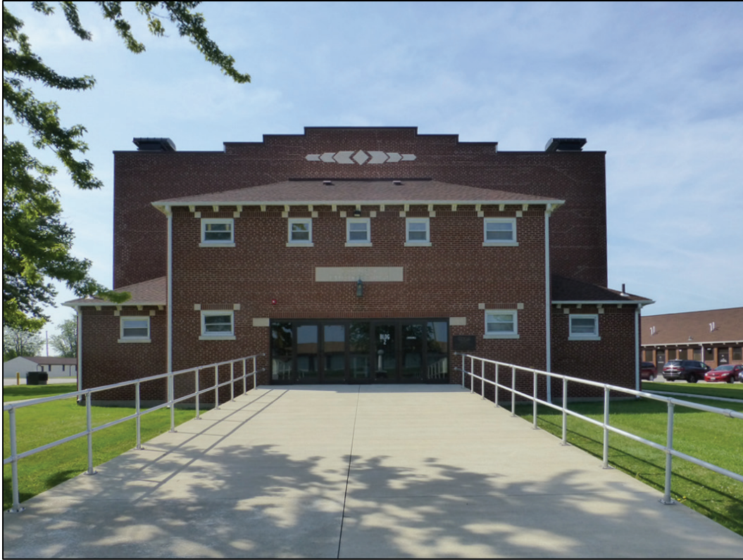
Figure 7. North side of Building 2 (ERDC-CERL 2017),
