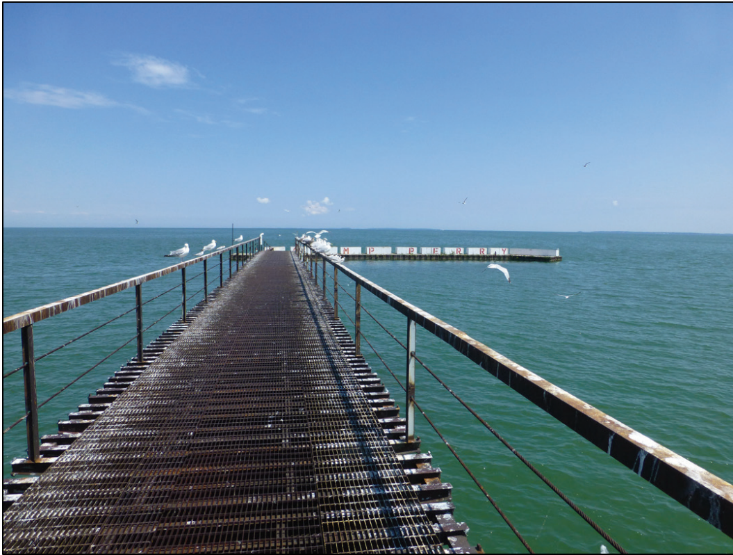
Figure 210. View north of bridge toward breakwater (ERDC-CERL 2017).
