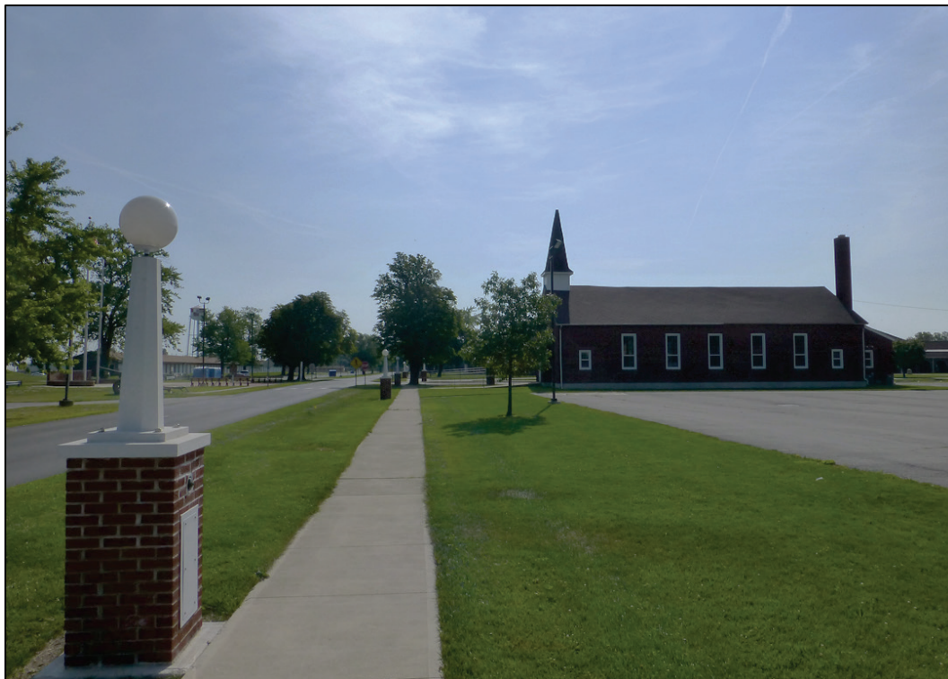
Figure 249. Looking east along Lawrence Road towards the chapel with a reconstructed 1936 street lamp on the left in Area I (ERDC-CERL 2017).
