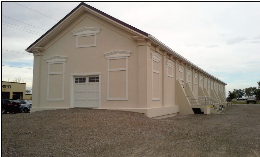
Figure 61. Looking south at Building 2009 (Camp Perry 2017).
