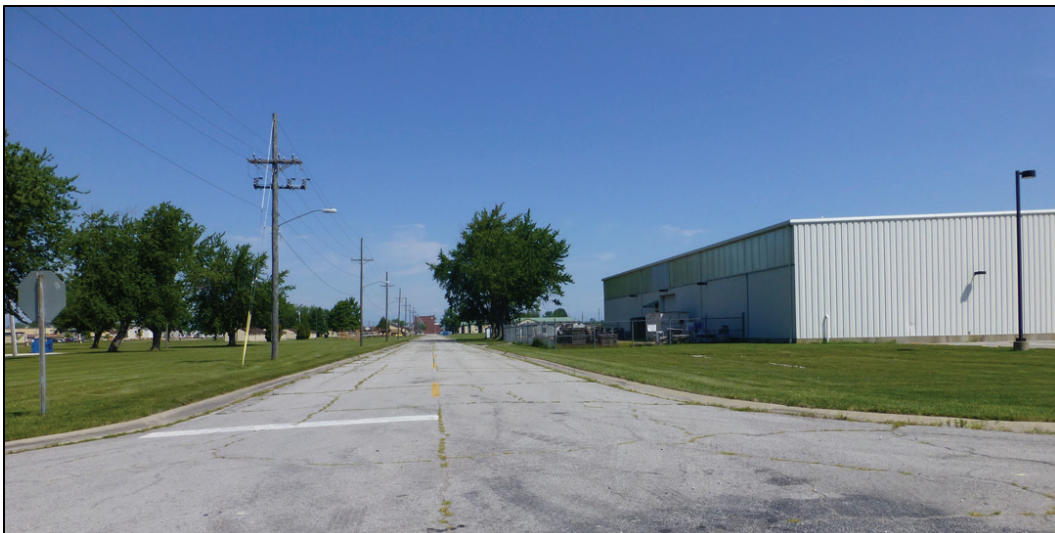
Figure 93. Looking north, with Building 3300 on the right (ERDC-CERL 2017).
