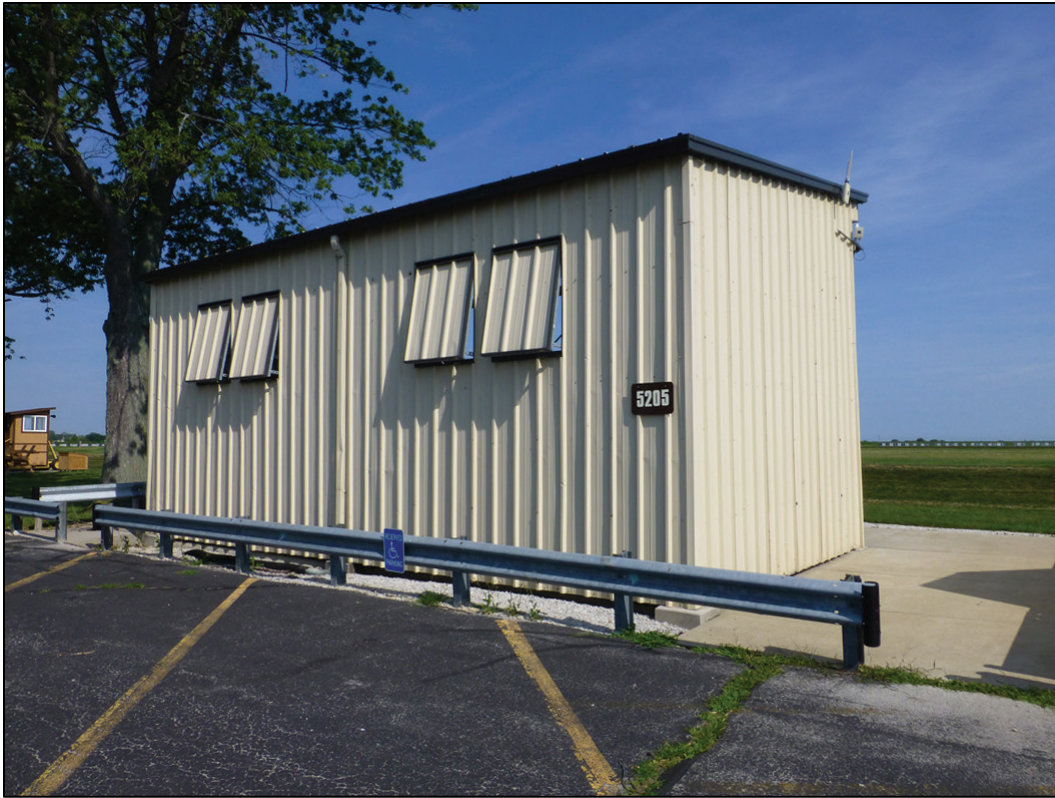
Figure 295. Looking north at Building 5205 in Area O (ERDC-CERL 2017).
