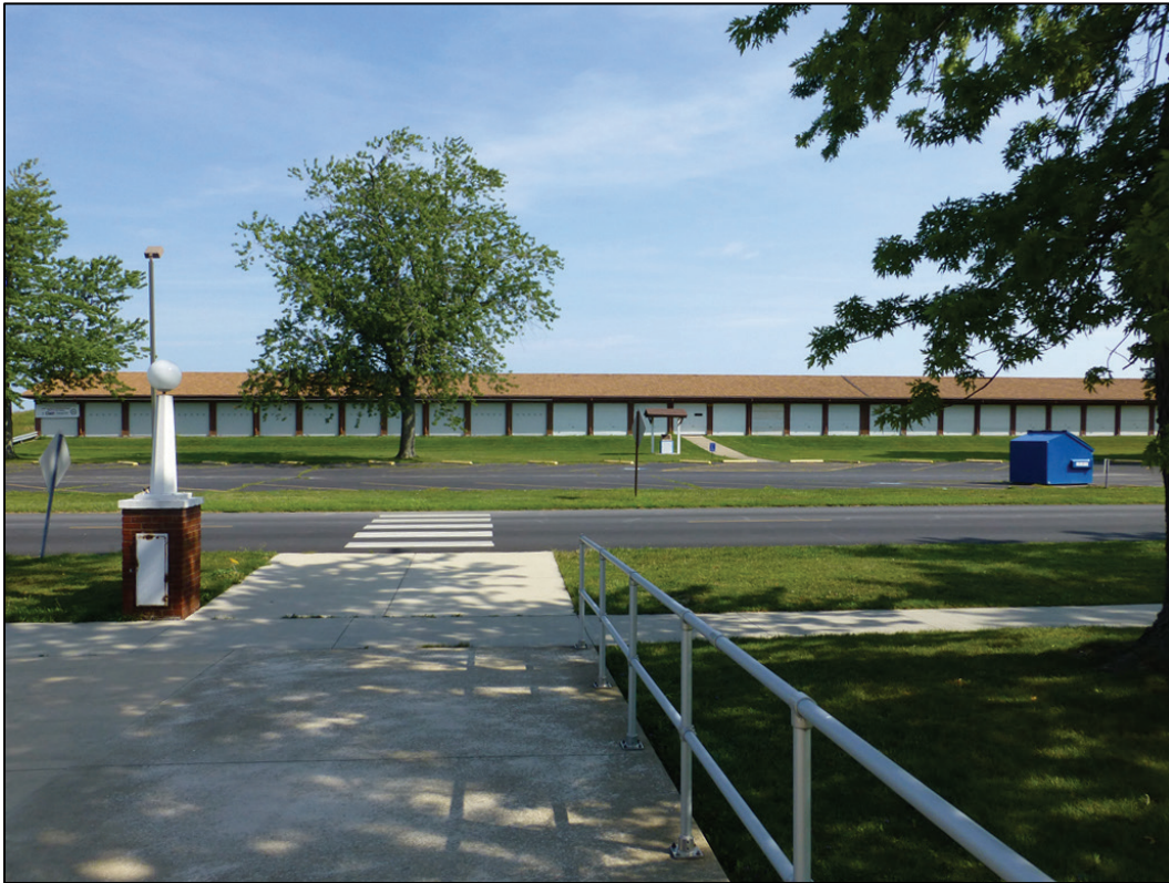
Figure 333. View north from auditorium entrance to firing range is now blocked by Building 5039 (ERDC-CERL 2017).
