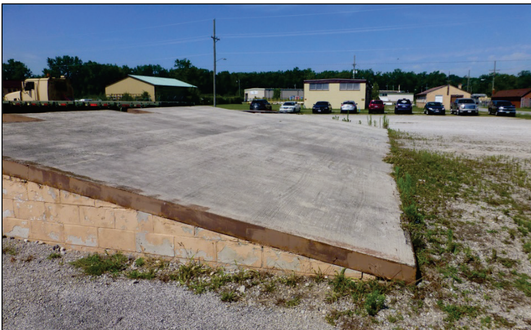
Figure 111. Looking east at the loading dock (ERDC-CERL 2017).
