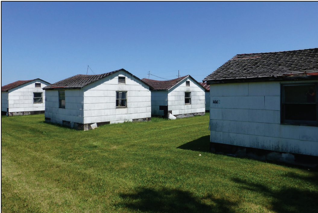
Figure 108. Looking northeast toward hutments KK 2-4, LL 2-4, and MM 2-4 (ERDC-CERL 2017).
