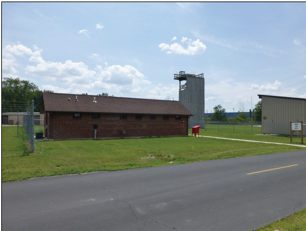
Figure 288. Looking south into Area N (ERDC-CERL 2017).
