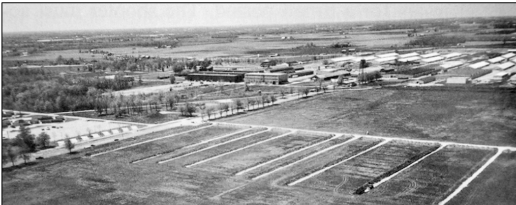
Figure 302. Young and Viale Ranges after drainage tiles were installed, no date (OHARNG).
