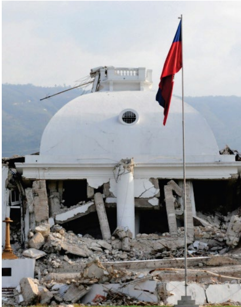
Figure 6. The Collapsed Presidential Palace of Haiti
