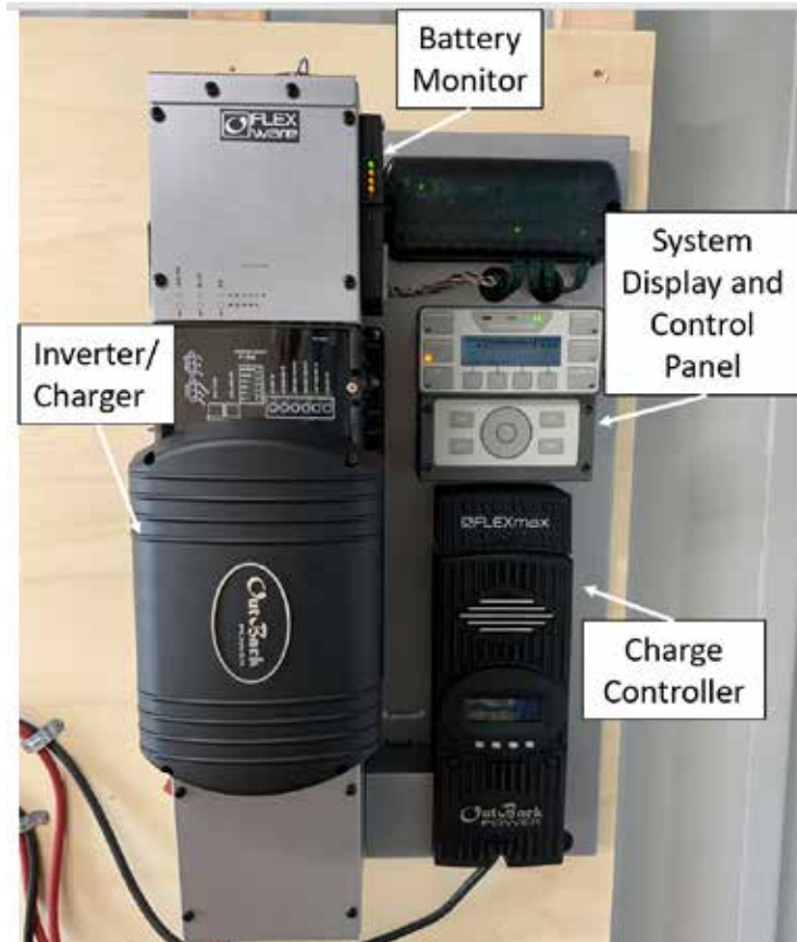
Figure 34. Microgrid Control System
