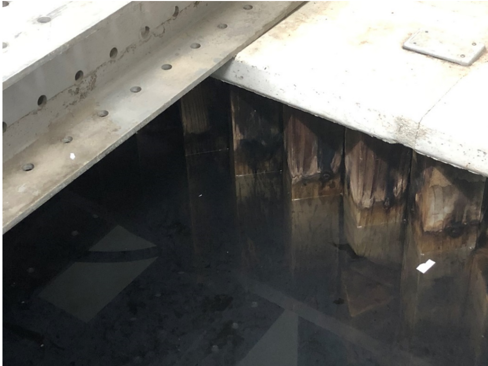
Figure 4. Non-reflective wall design
