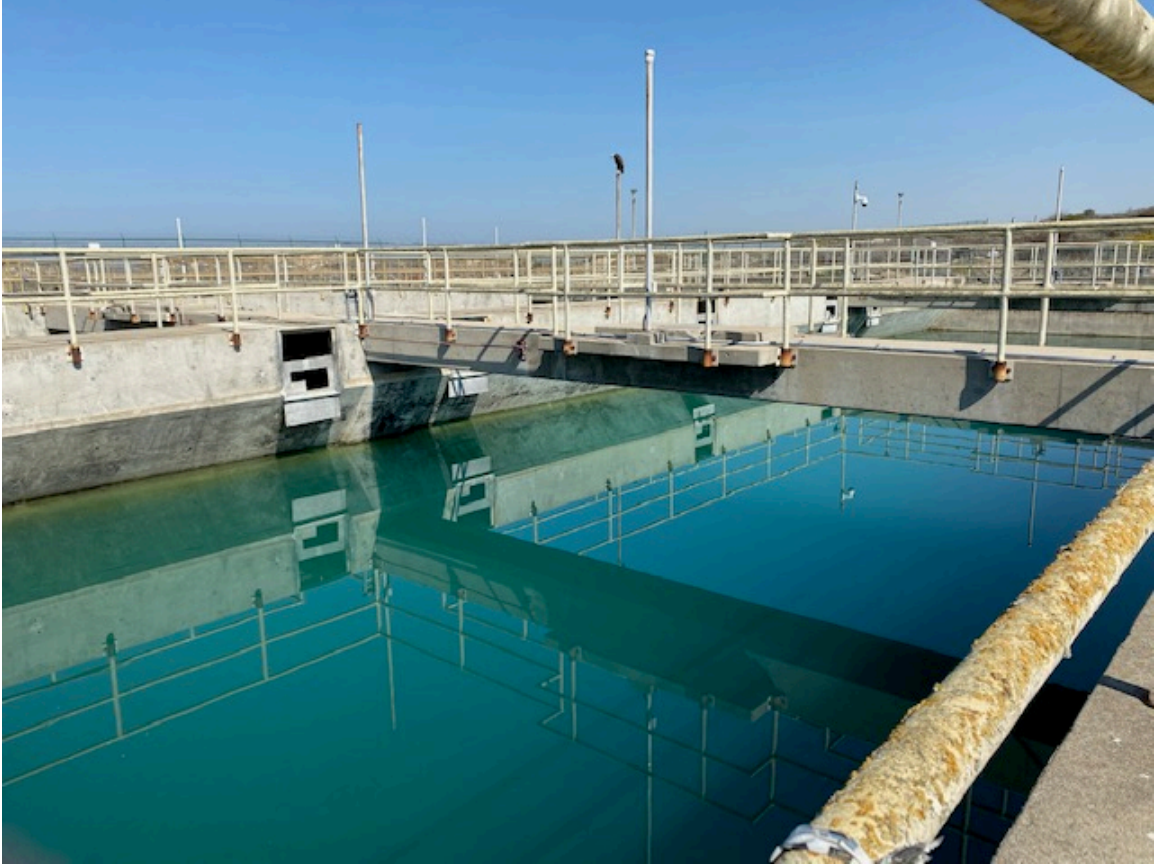
Figure 28. Tank AQ1 with catwalk
