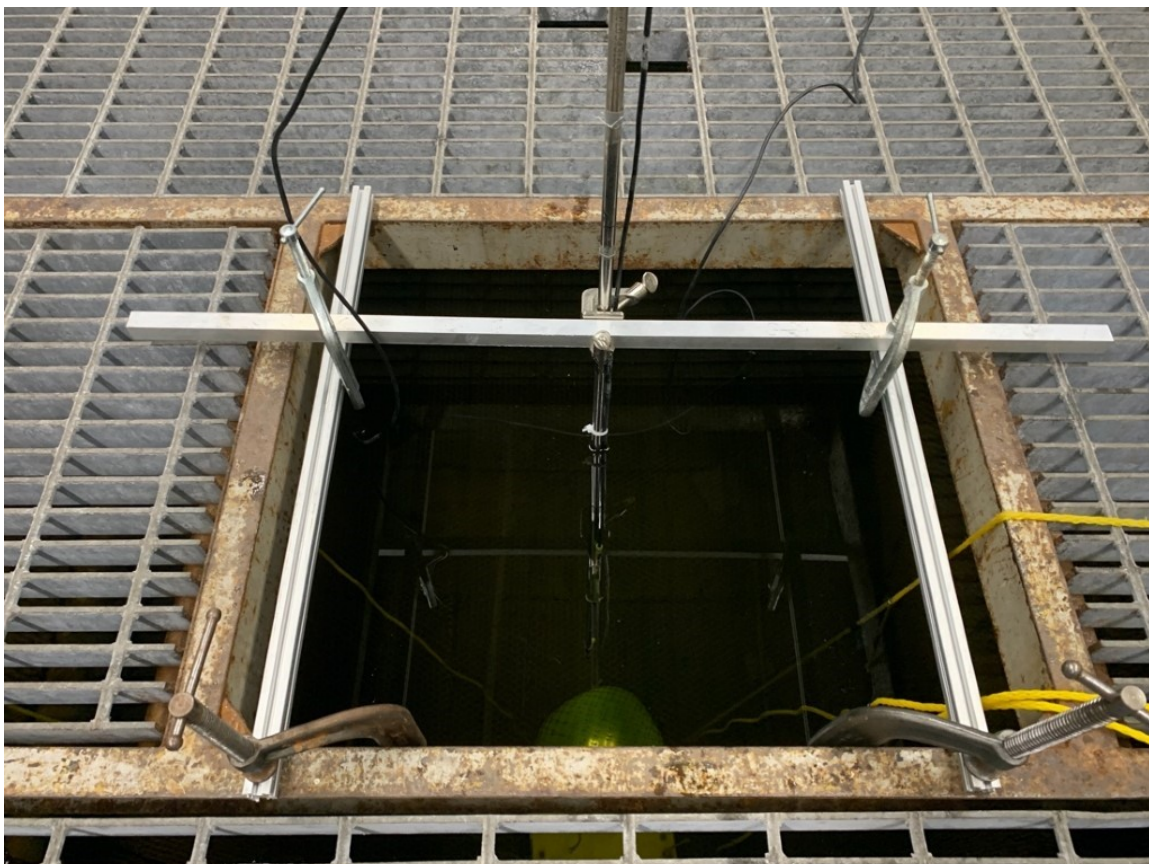
Figure 16. Projecting hydrophone structure
