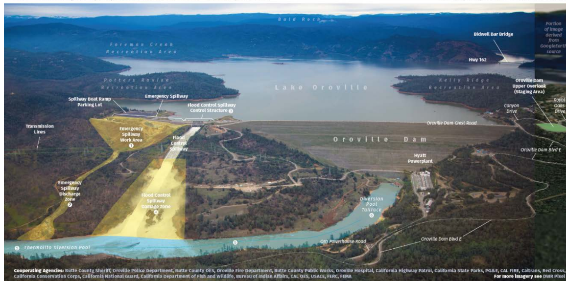
Figure 4. Oroville Dam Overview 109
