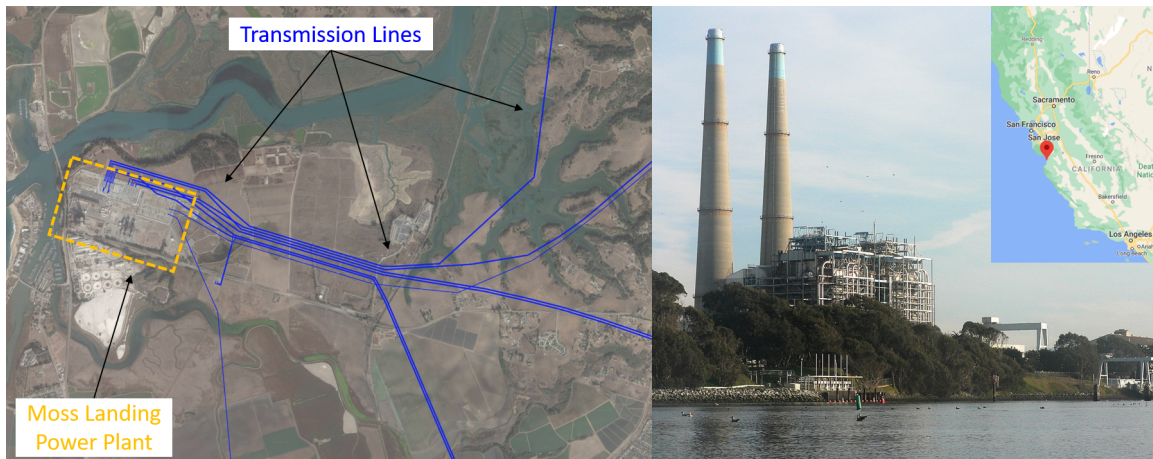
Figure 3.4. Moss Landing Power Plant. The natural gas powered electricity plant located in Moss Landing is an example of one of the many generation plants in the state of California utilized by PG&E. The satellite map (left) shows where the transmission lines start. Some of the areas they carry electric power to are Santa Cruz to the north and Monterey/Salinas to the south. (left) Adapted from Pacific Gas & Electric Company (2019a). (right) Source: Google Maps and Wikipedia (2020).
