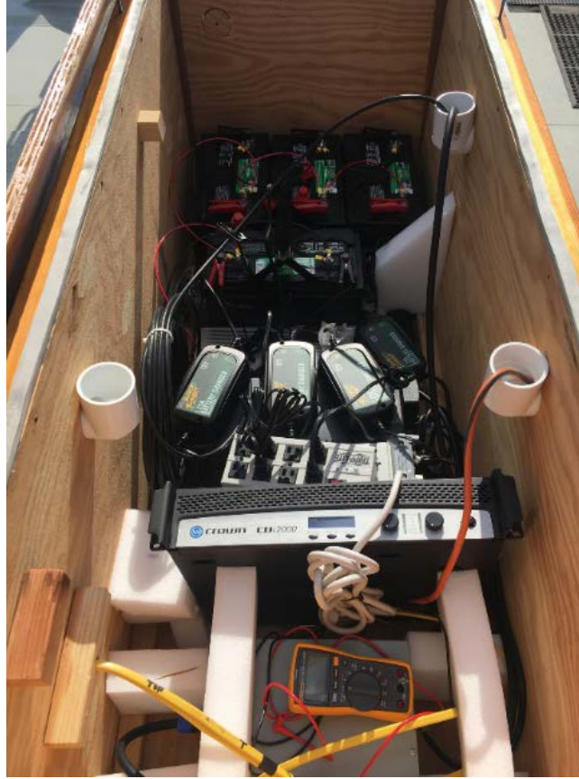
Figure 11. Electronic equipment inside the coffin which powered and delivered the signal to the source.
