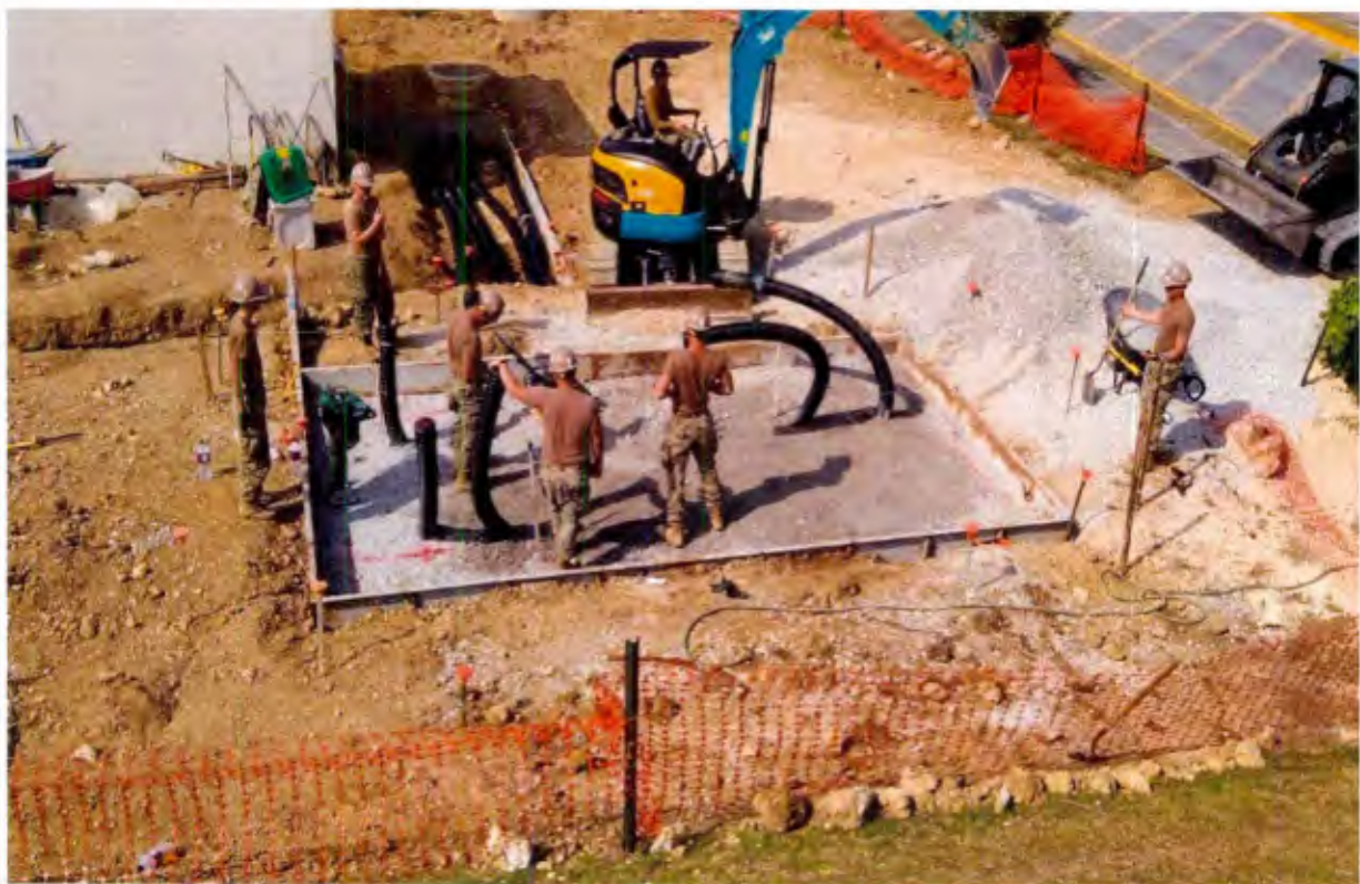
Figure 5.2.2. Seabees working to install the conduits and concrete pad.
