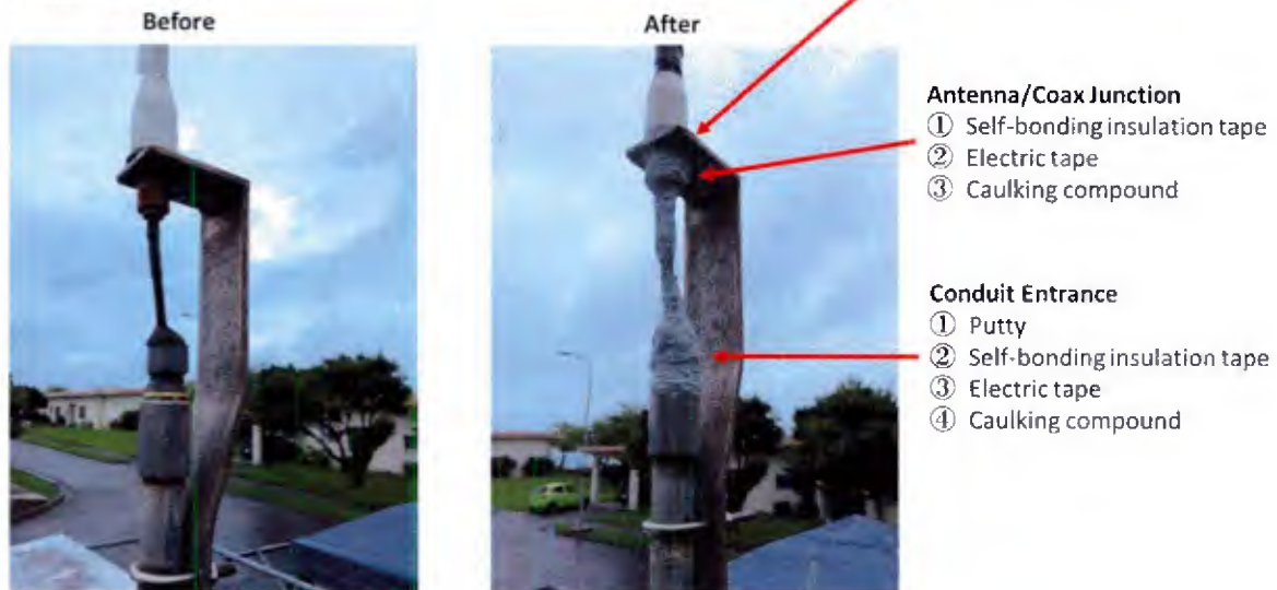
Figure 5.2.5. Example of the antenna replacement work.
