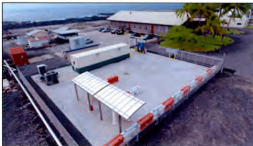
Figure 2.4.1. HNEI NELHA hydrogen station.
