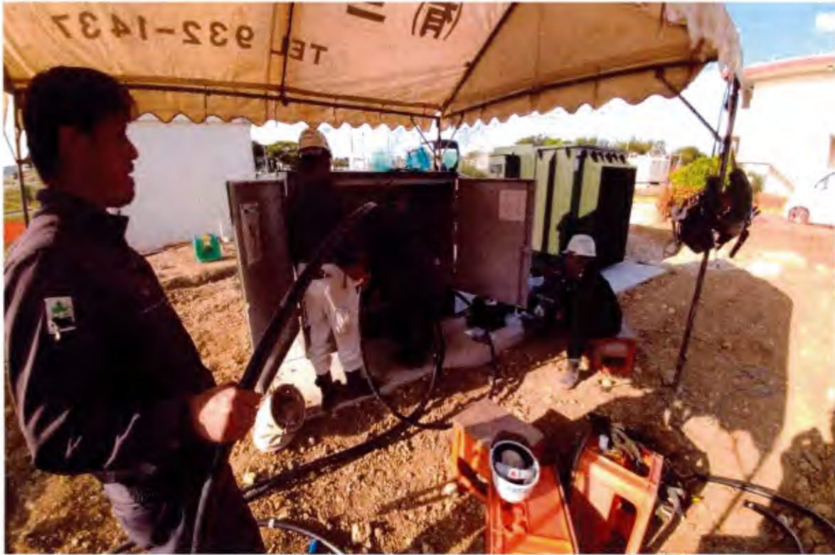
Figure 5.2.3. HNEI's electrical contractor installing the electrical cables and terminations.
