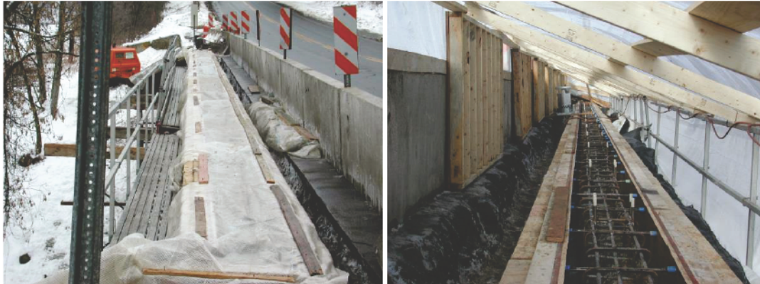
Figure 1. Bridge curb repairs performed in the winter of 2002, on the west and east sides of the Trues Brook Bridge in Lebanon, NH. The west side (left) of the bridge was repaired using CWAS concrete, while the east side (right) was repaired using conventional concrete in a heated enclosure.
