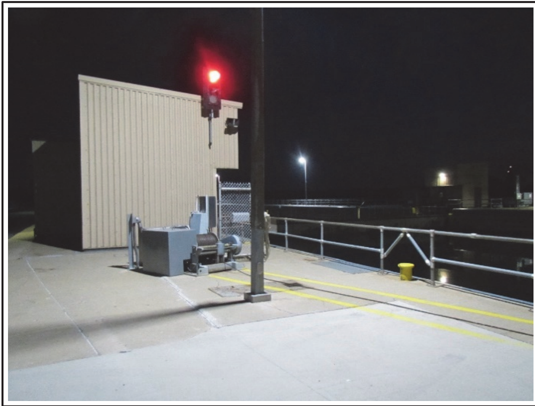
Figure 36. Hydraulic tow haulage unit at Lockport Lock.
