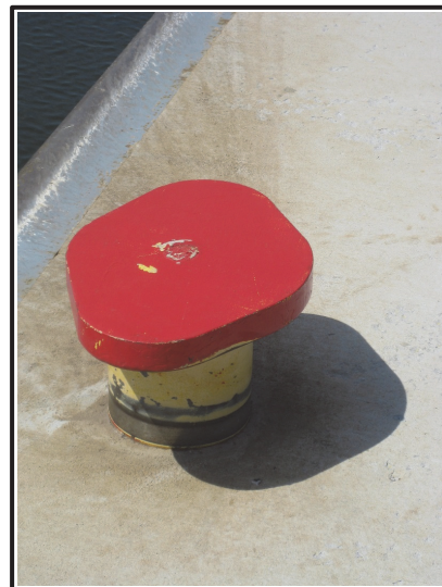
Figure 26. New mooring bit.
