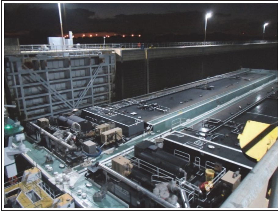
Figure 45. Lower miter gates lighting improvement at Lockport Lock.
