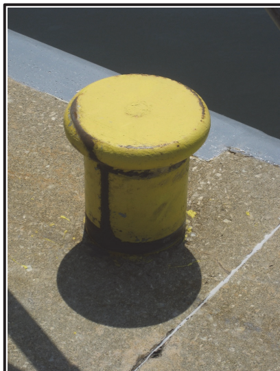
Figure 25. Old mooring bit.
