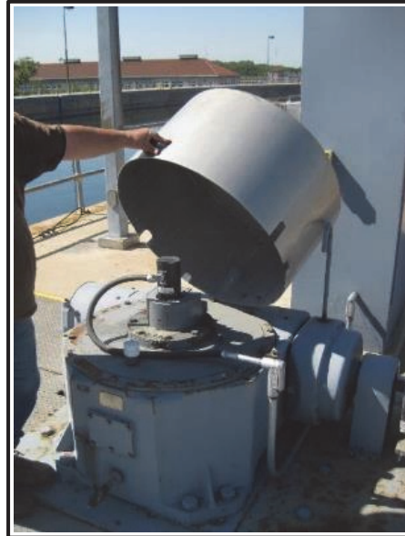
Figure 3. Gearbox cover at Lockport Lock.
