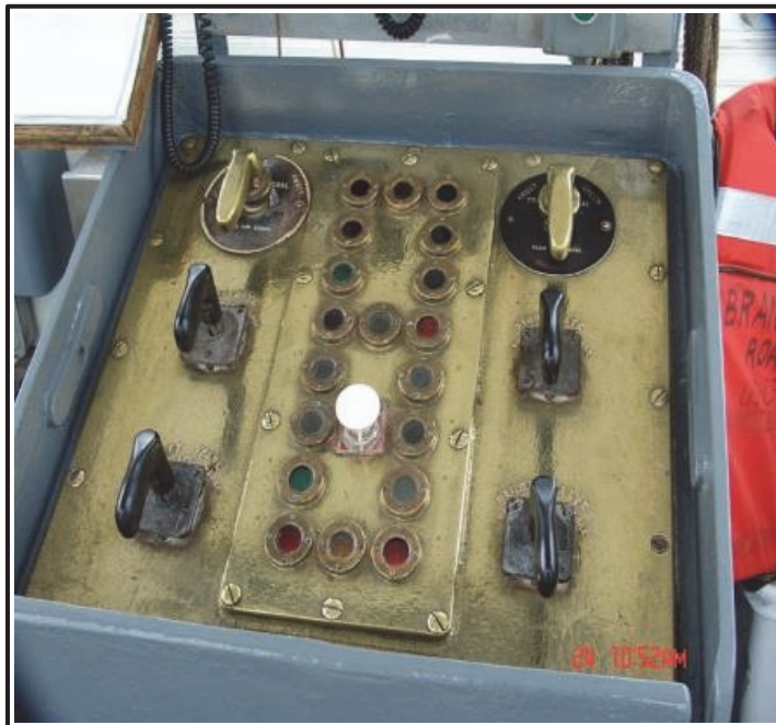
Figure 14. Brandon Road control panels.
