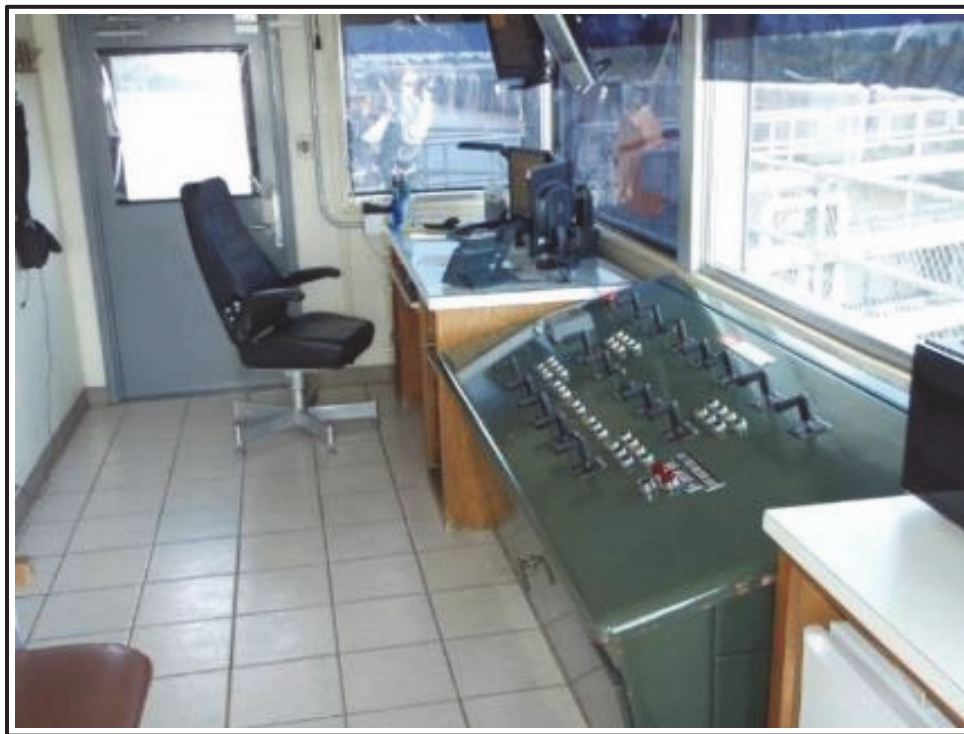
Figure 12. Pre-renovation Port Allen control room.
