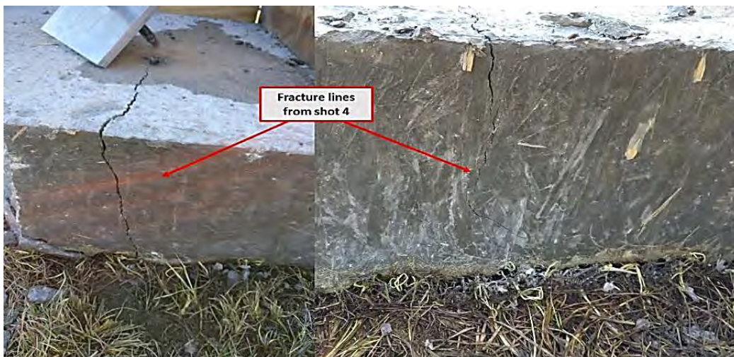
Figure 92. Shot 4: Fracture Lines in Concrete Test Slab 1
