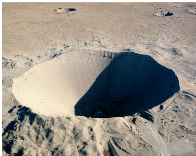
Figure 6. Sedan Crater at Nevada Test Site Excavated by a Plowshare Test
