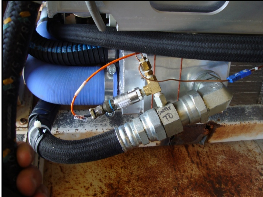
Figure A-3. Thermocouple and pressure transducer measuring oil temperature and pressure into transmission cooler.
