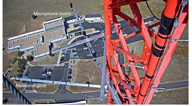
FIG. 3. (Color online) Microphone and meteorological booms attached to the tower (view from the tower towards the ground).
