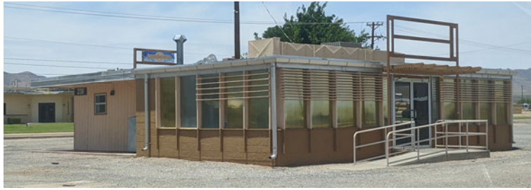
Figure 60: Simple 1 Viewed from the Ground
