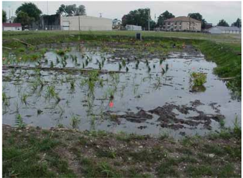
Figure 1: Artificial wetland system constructed by ENV for the cleanup of a groundwater plume of tetrachloroethylene located at Wright-Patterson AFB.
