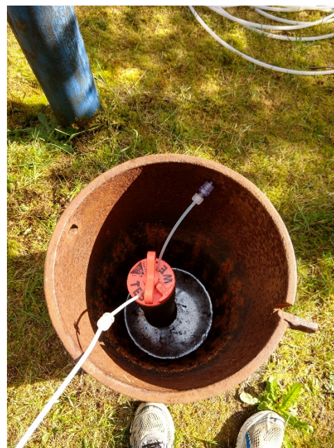
Figure 12. Well Cap Sealed in Place with Sparge Line and Check Valve
