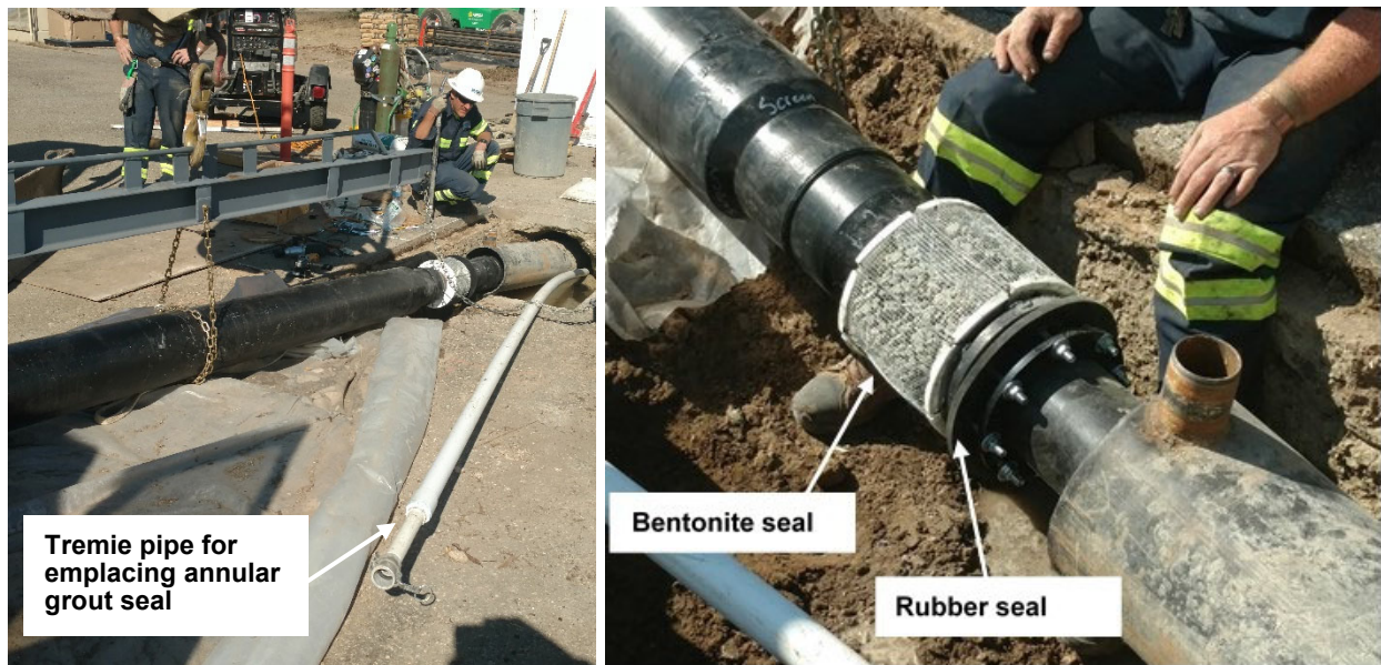
Figure 24. Treatment Media Cartridge Installation
