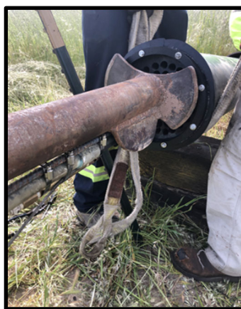
Figure 25. Monitoring Cartridge Installation
