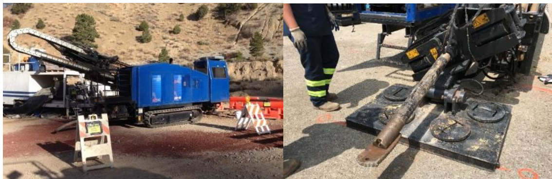
Figure 20. Directional Drilling Rig and Drill Bit
