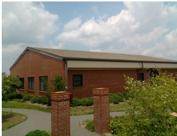
Figure 9. Ft. Bragg Building 3-2232 where the Energy Efficient Phase Change Materials (PCM) Insulation was demonstrated
