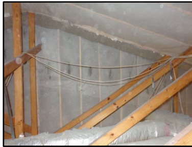
Figure 18. Phase 2 cellulose insulation
