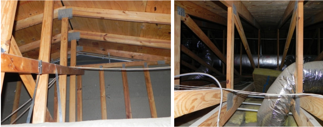
Figure 6. View from attic of Demonstration Bldg. at Ft. Bragg. Left: Cellulose insulation is to be blown in to adhere to the roof deck. Right: HVAC ducts run through the attic.
