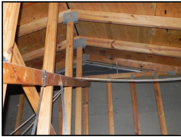
Figure 17. Phase 1 uninsulated attic
