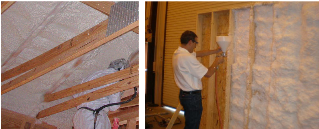
Figure 7. Typical application of blown-in cellulose insulation
