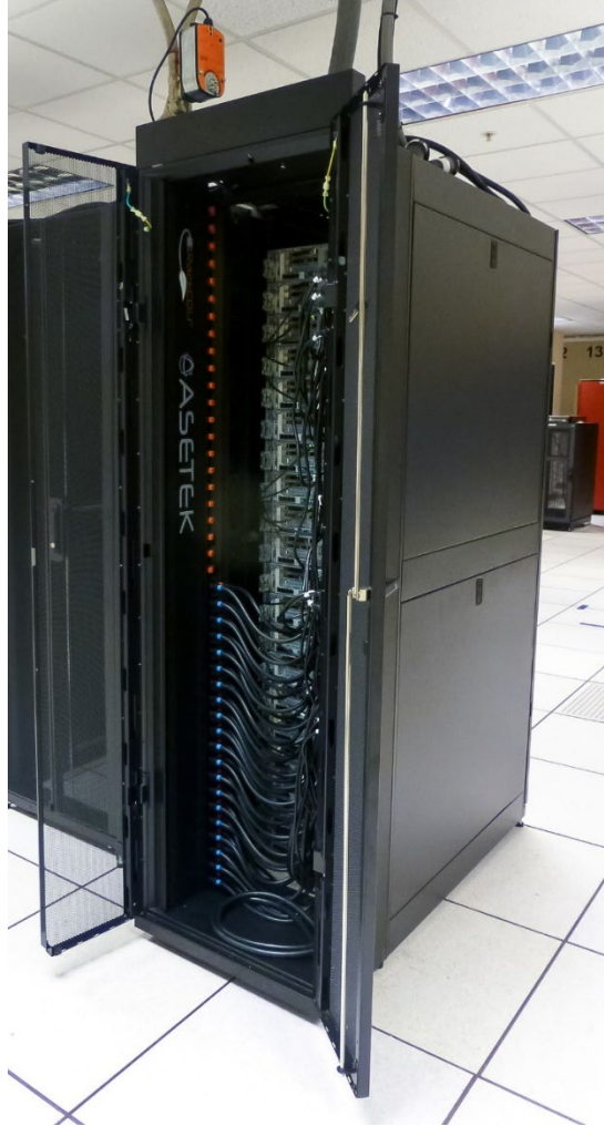
Figure 10. Rear View of Phase 1 Rack Installed at Redstone
