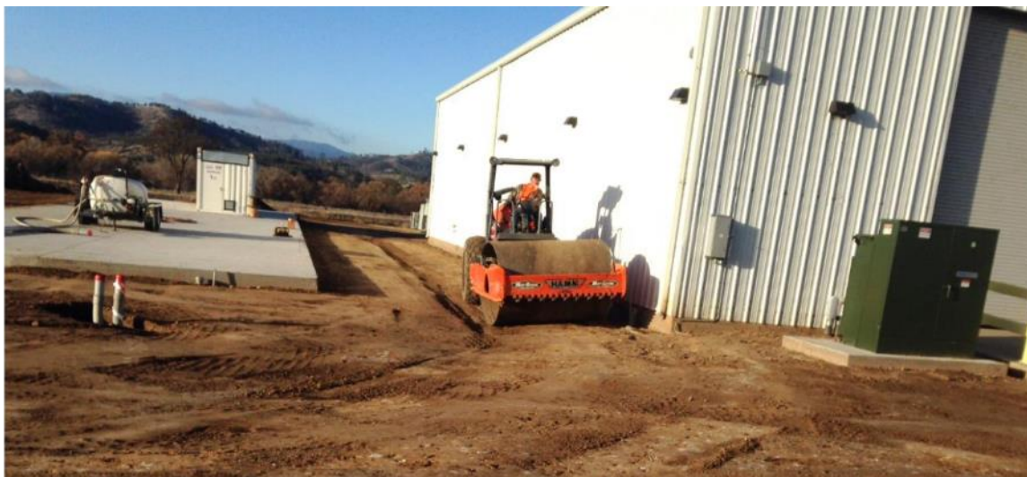
Figure 5. Site Preparation Work in 2016
