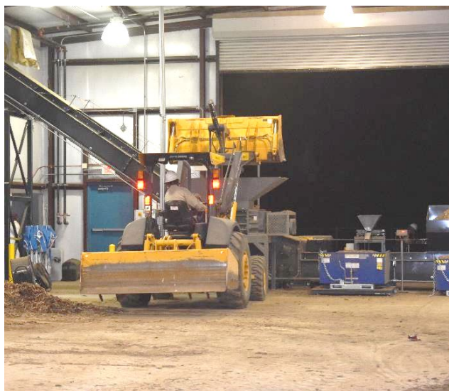
Figure 8. Feed Operator Shredding Waste Wood Feedstock in Bldg. 339.
