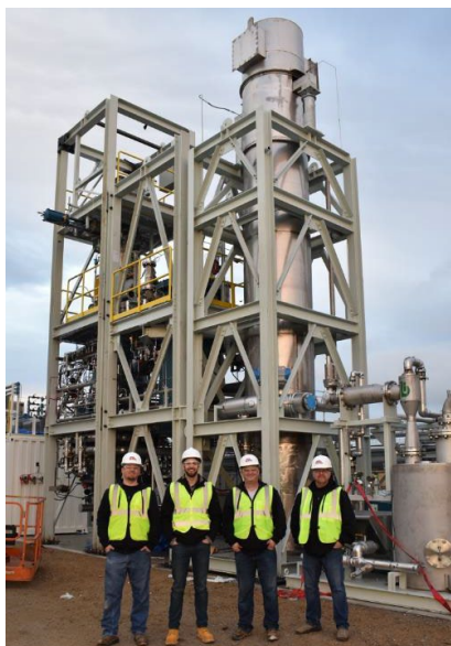
Figure 2. Sierra Energy's Gasifier, Polisher & Recuperator Nearing Mechanical Install Completion in 2017
