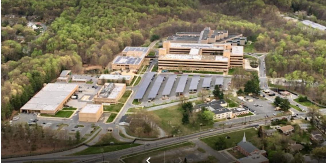
Figure 2: Army Research Center NSRL Building, Adelphi Maryland
