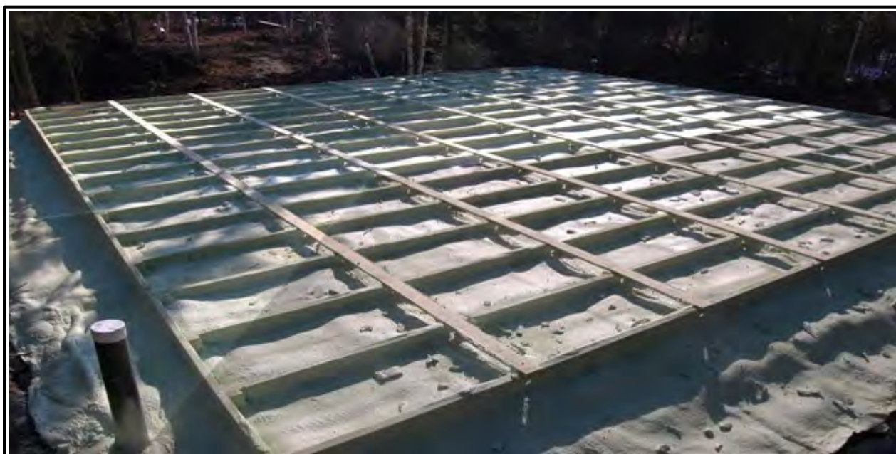
Figure 64. Raft foundation as it was being installed under one of the two Sustainable Village homes.
