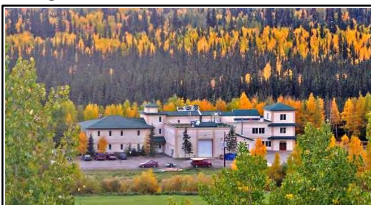
Figure 54. CCHRC RTF with the addition built in 2013.
