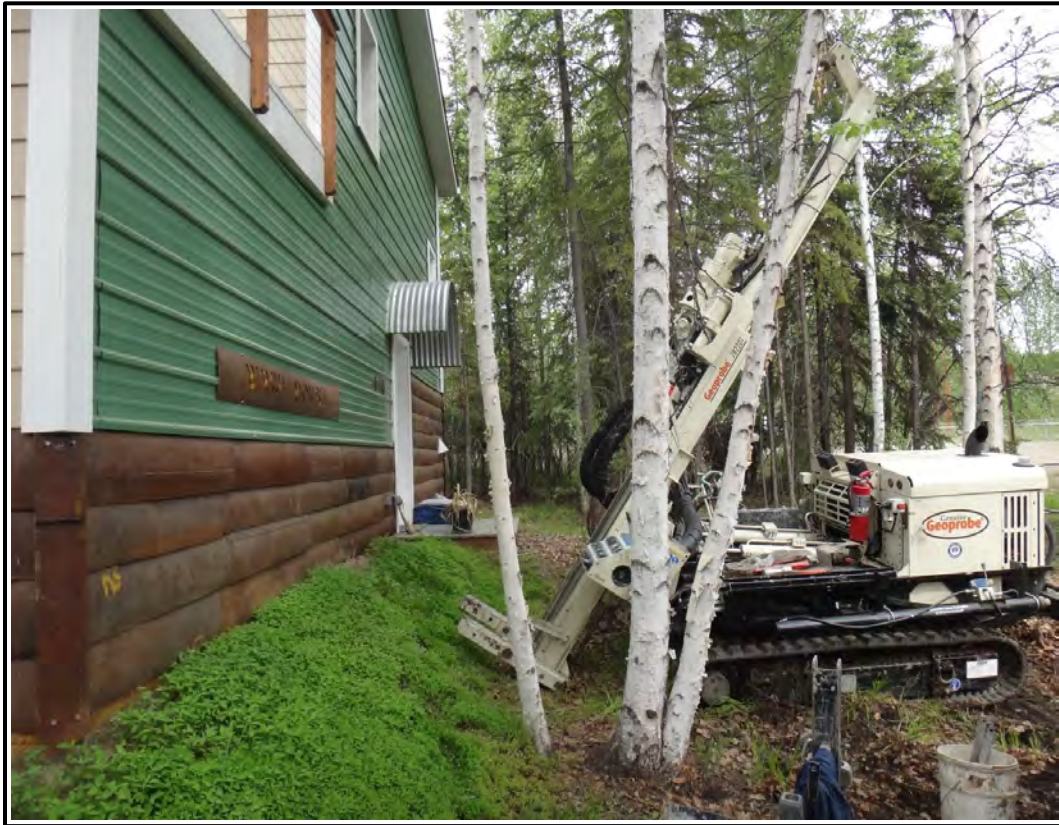
Figure 77. A directional drilling rig. Drilling a sensor tube hole under an existing house at the Sustainable Village at UAF.
