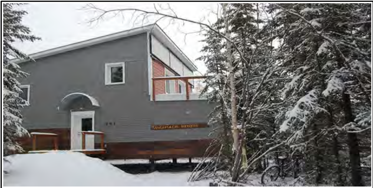
Figure 62. One of the two Sustainable Village homes on pile foundations installed on permafrost ground.
