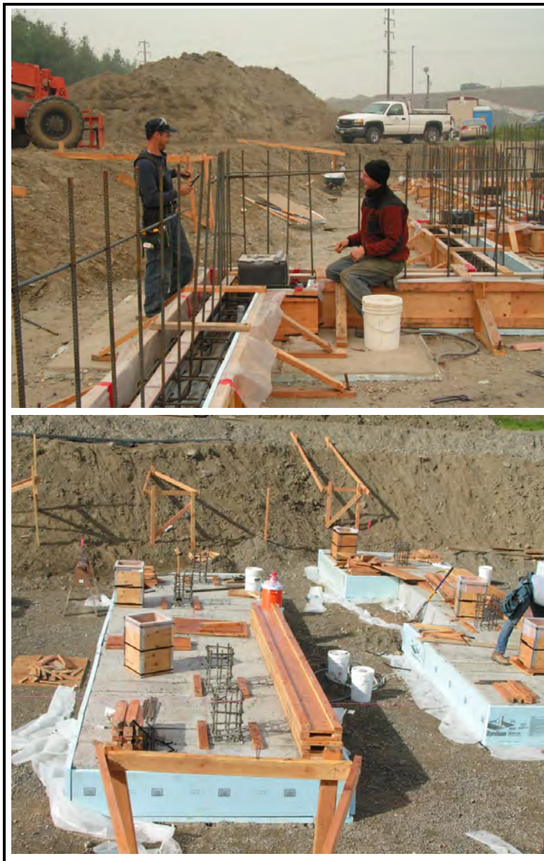
Figure 76. Preparing the foundation for concrete pouring. The white buckets are full of sensor wires. The sensors are already in the conduit in the ground. The wires are in 1-in. Loctite conduit running back to the buckets. The buckets make the wiring more visible to the building crew.
