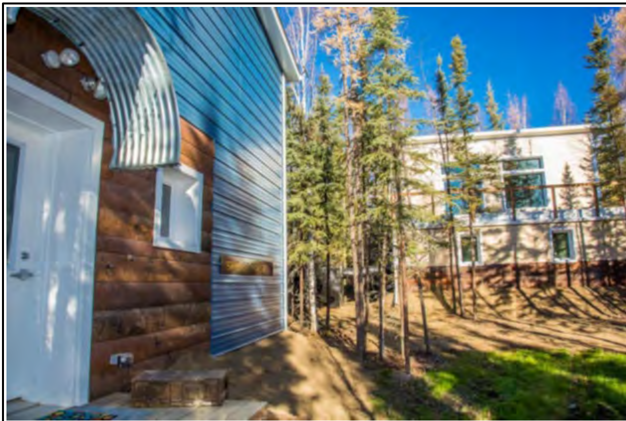
Figure 63. The two Sustainable Village homes on the insulated raft foundations installed on the ground.
