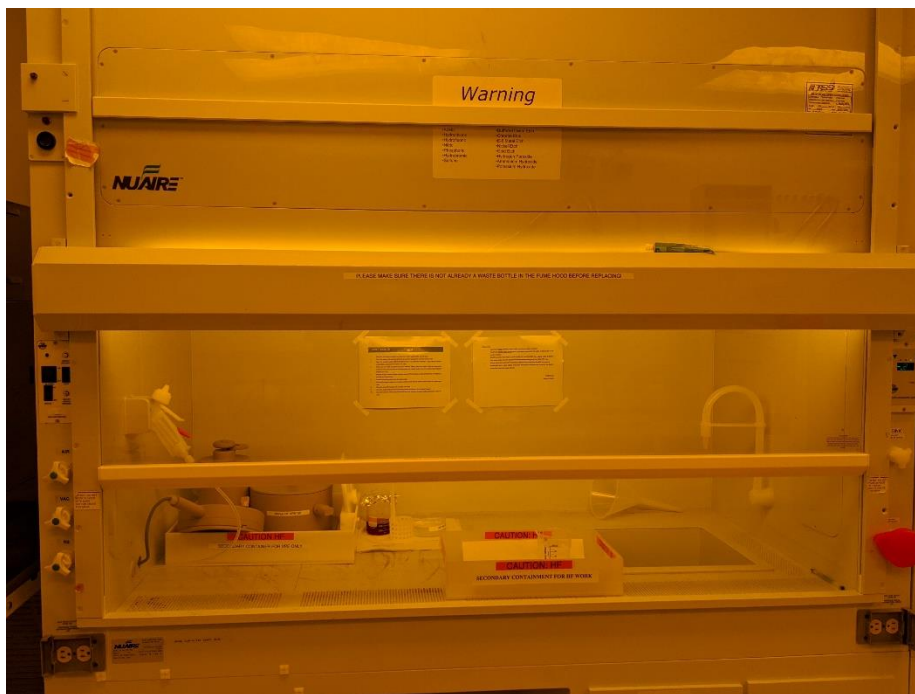
Figure 45. Polypropylene fume hood with secondary container for working with hydrofluoric (HF) acid and buffered oxide etchant (BOE).
