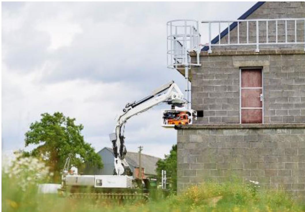
Figure 1-12: Large Unmanned Ground Vehicle Deploying the Small Unmanned Ground Vehicle on the Top of a Building.
