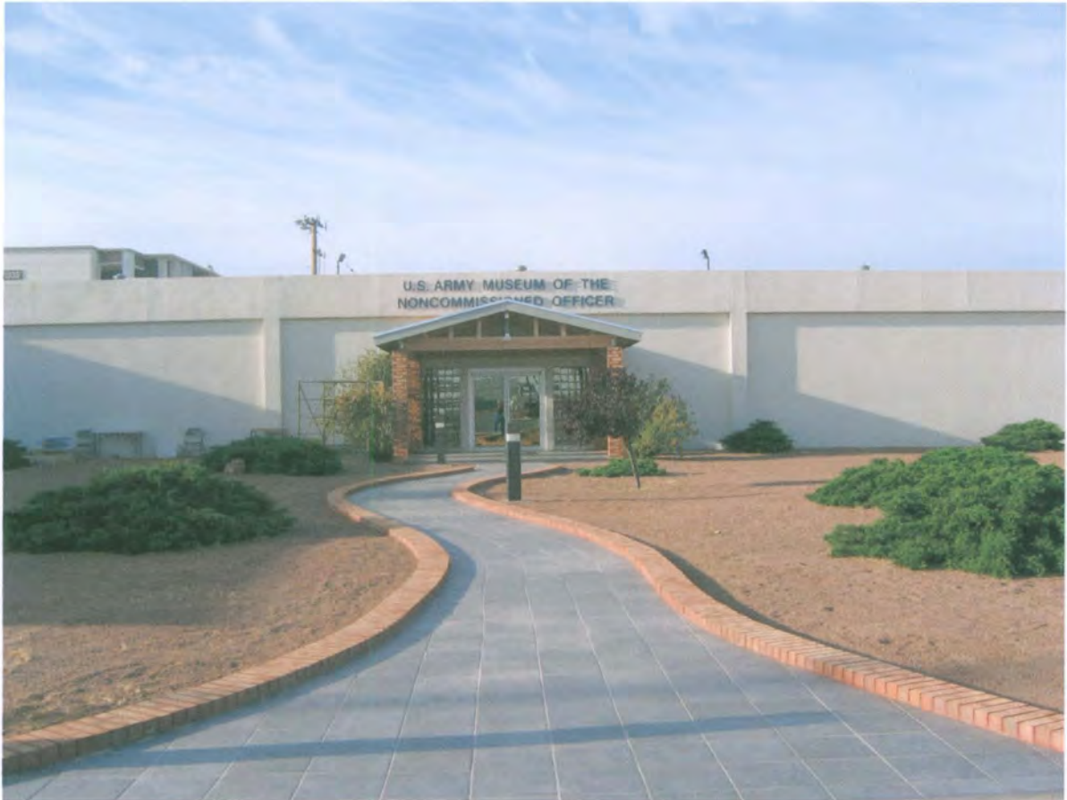
New Tile Walkway and Portico at the NCO Museum.
