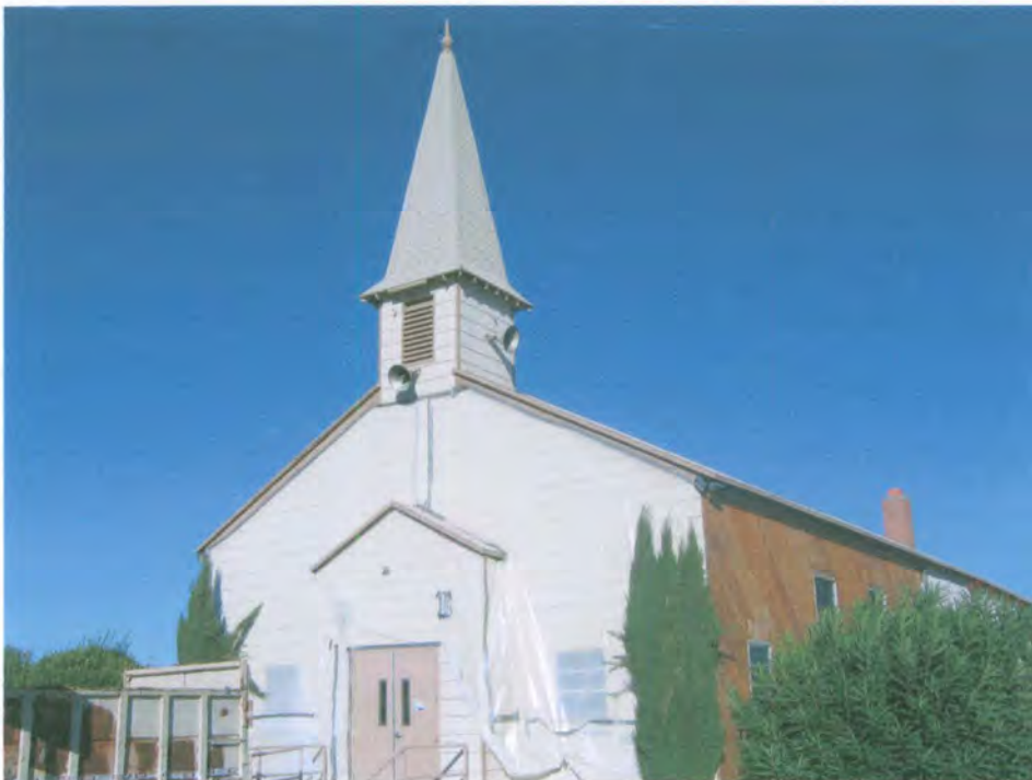
Biggs Chapel, December 2005, in Midst of Asbestos Removal
