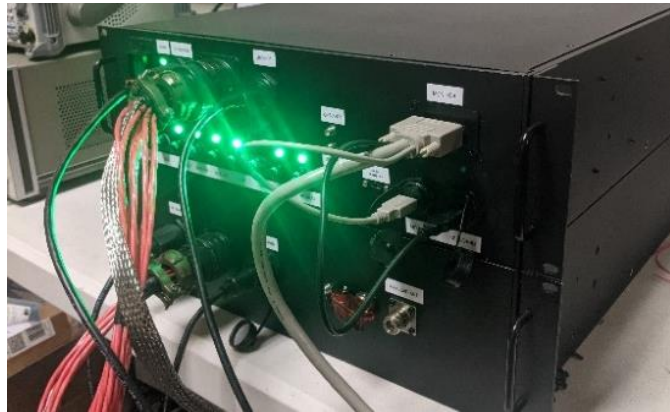
Figure I-3: SPHINX Payload Chassis 2 - Power Distribution Board
