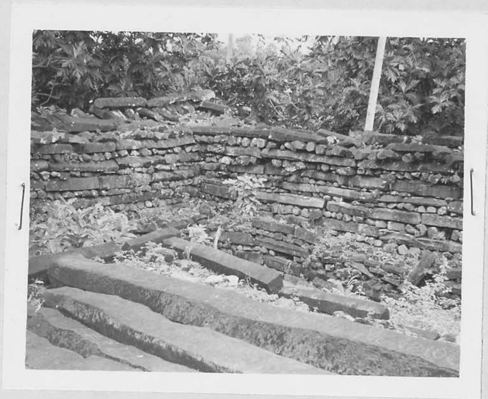
Illustration 11: Nanmadol construction using columnar basalt natural crystals as "stone logs" 1-2' thick and 10-15' long.
