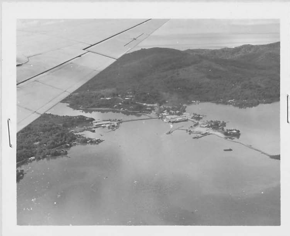
Illustration 1: Town of Colonia on Yap located on western side of Tomil Harbor. View is looking north-west.
