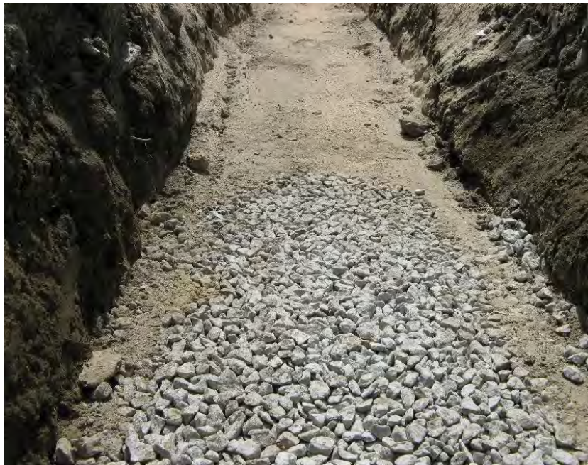
FIGURE 3.4: Transition between gravel and sand in-trench
