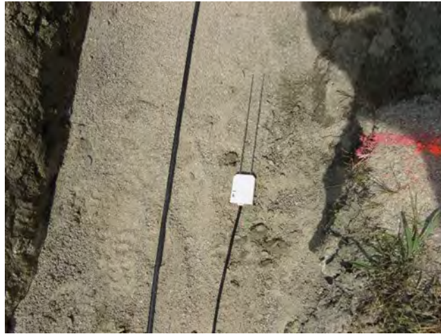
FIGURE 3.6: Placement of CS650 sensors relative to the fiber optic cable
