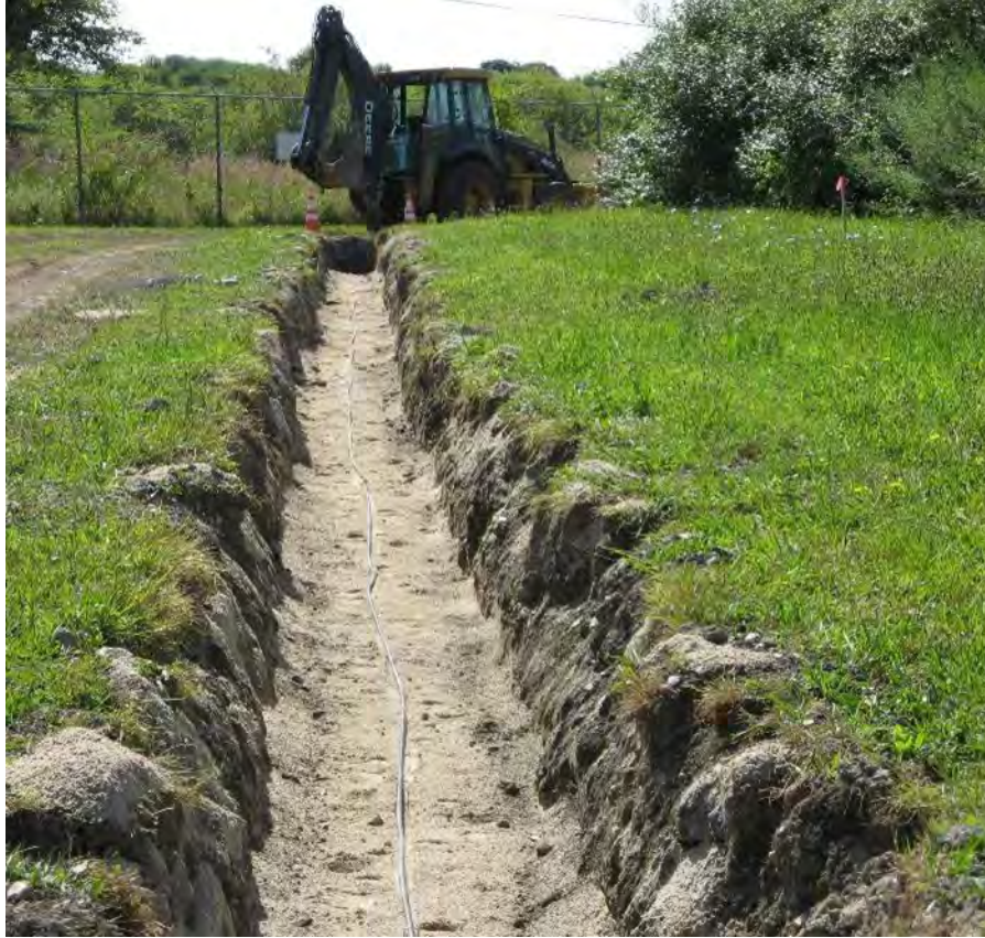
FIGURE 3.5: Fiber optic cable along the centerline of the sand trench.
