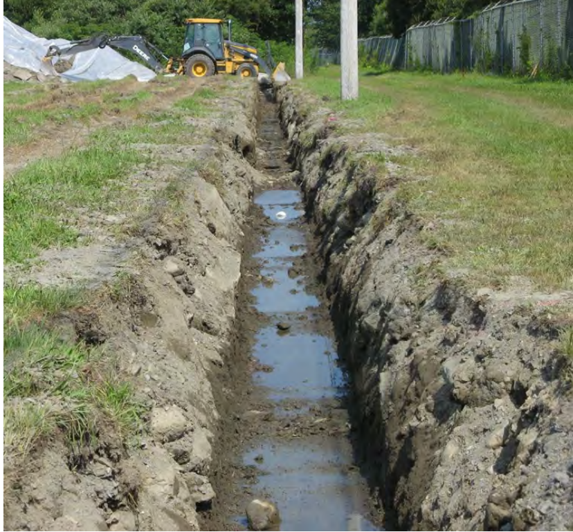
FIGURE 3.3: Complete excavated trench for flowable fill
