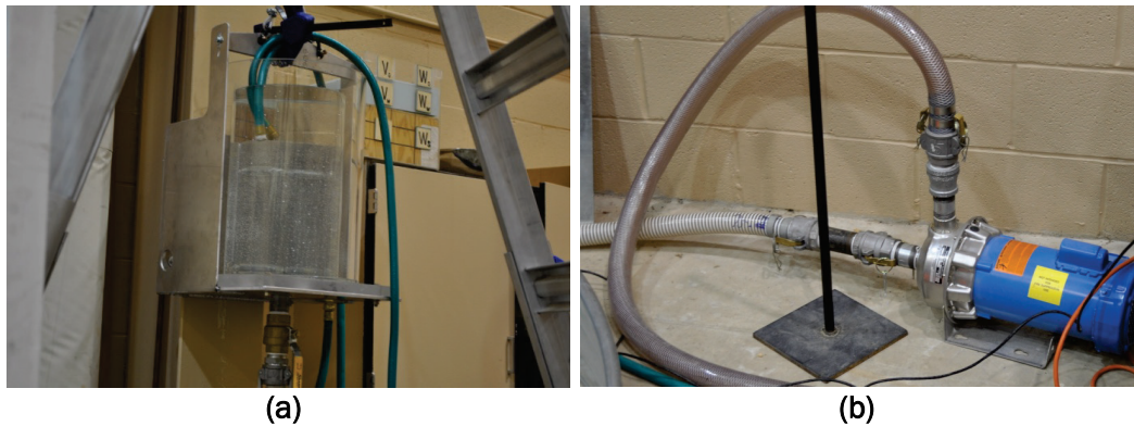
Figure 10. (a) Constant head tank with hose supplying water. (b) Pump with 3.81-cm (1.5-in.) tubes.
