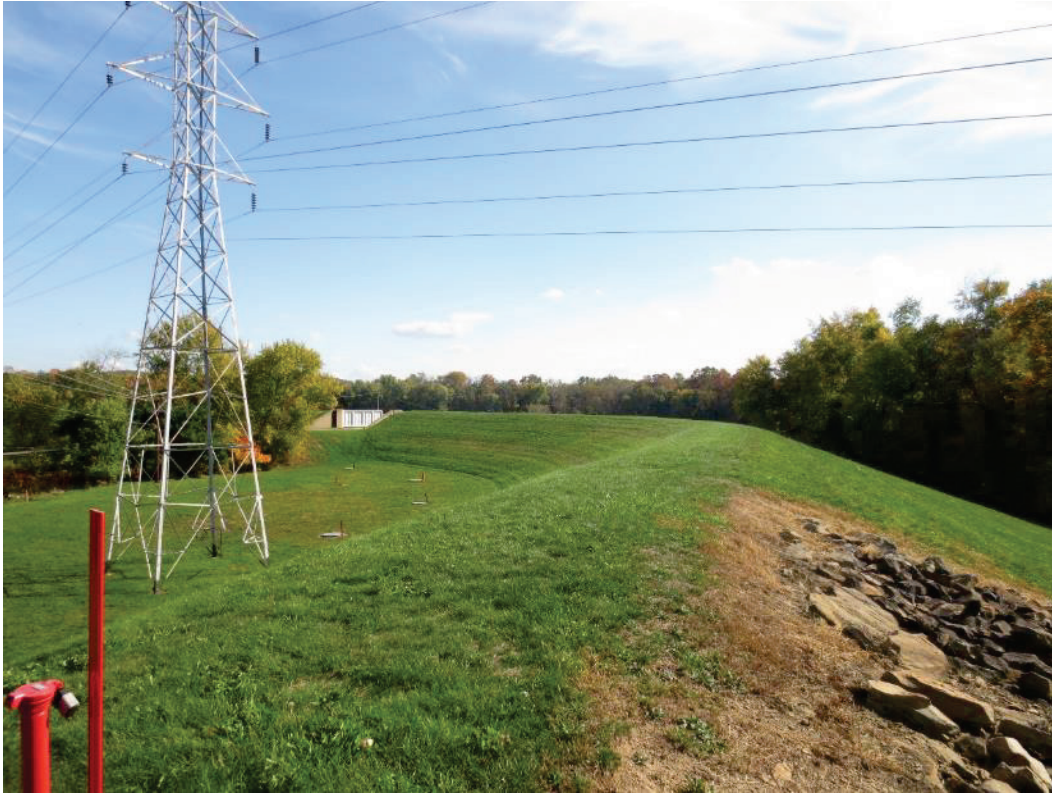
Figure 2. Looking south on the Magnolia Levee crest.
