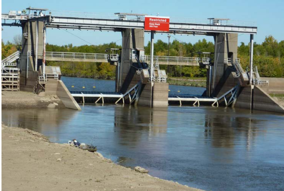
Figure 13. Site of third field test, Kaskaskia Lock and Dam, Illinois.
