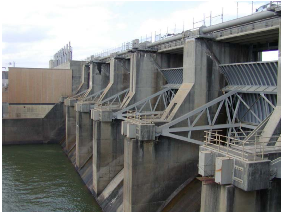
Figure 9. Typical tainter gates and trunnions.
