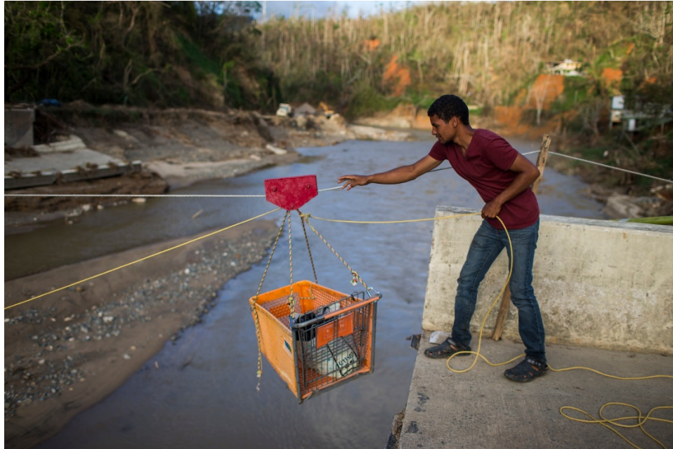
Figure 1. Pulley System to Span the Río Viví. 166
