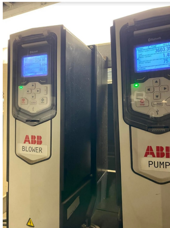
Figure 14. ORC Blower and Therminol Pump Interface
