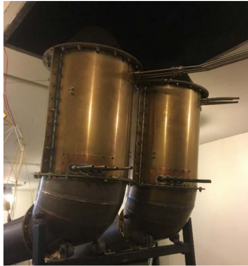
Figure 17. Kaim's Modified Heat Exchanger Installation. Source: [6].
