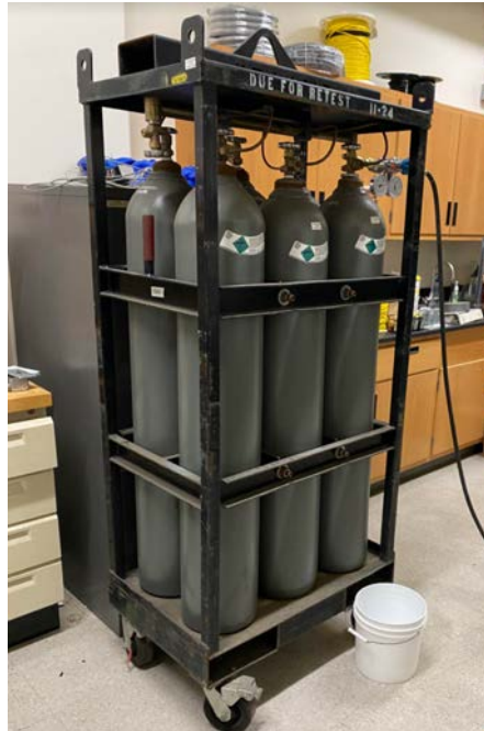
Figure 24. Compressed CO 2 Tanks
