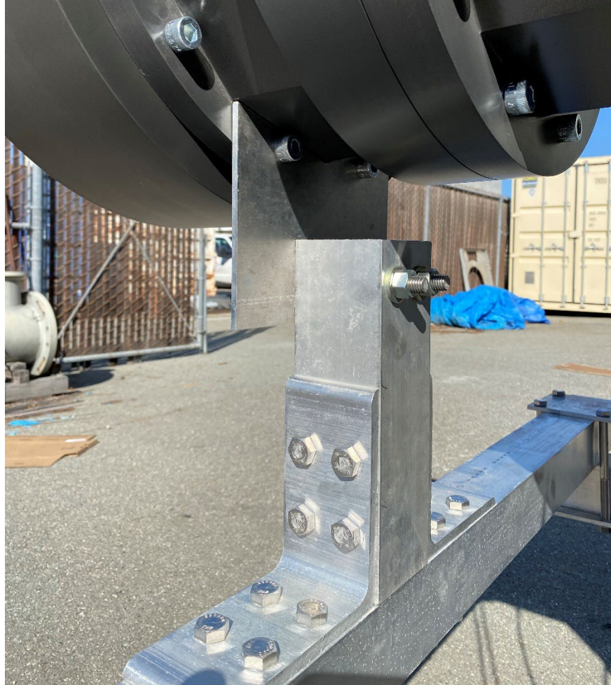
Figure 40. Bell mouth support after installation
