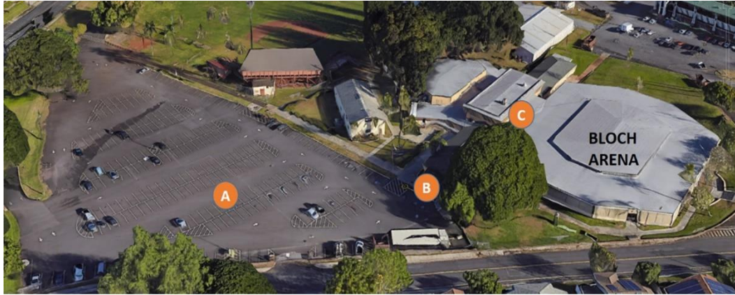
Figure 1. Bloch Arena and parking lot, top: aerial view, bottom: indoors.
