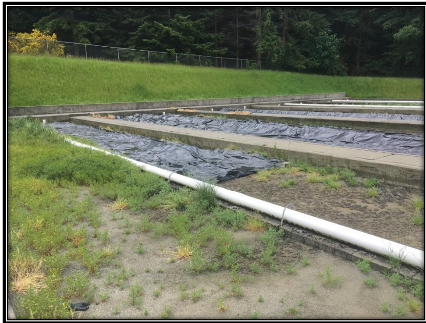
Figure 5-2: Aging Sand Filters at NAVMAG Indian Island
