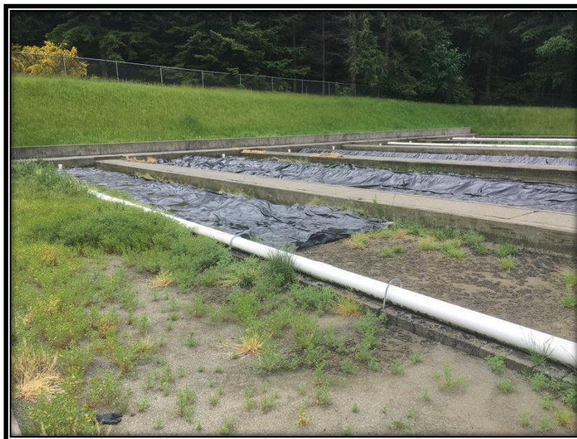
Figure 4-6: Aging Sand Filters at NAVMAG Indian Island
