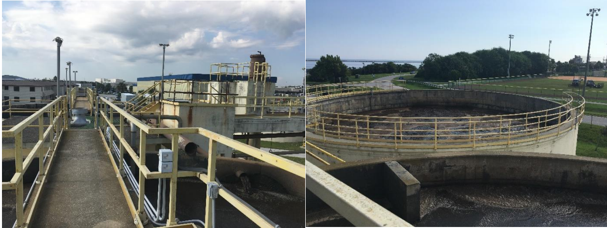
Figure 4-9 NAVSTA Mayport Wastewater Treatment Facility 2017.
