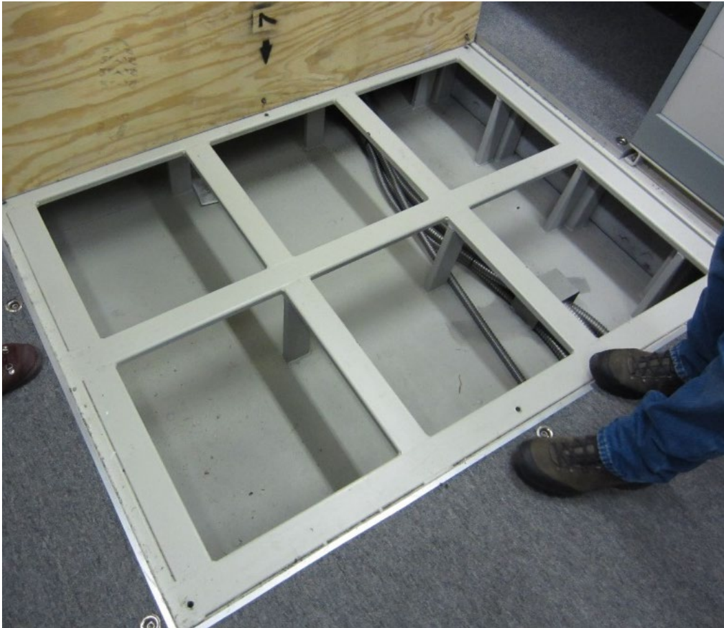
Figure 11. Photograph of the raised access floor framing.
