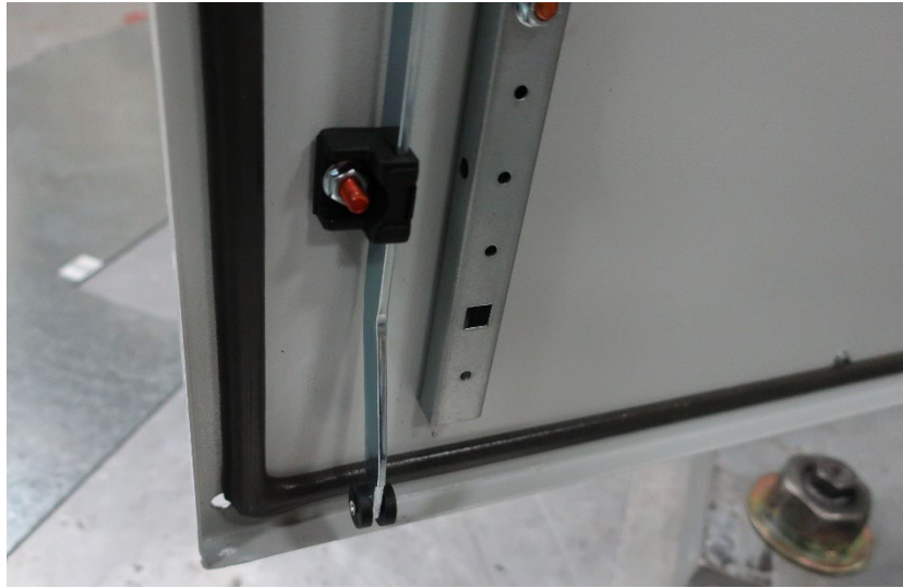
Figure 35. Bottom of vertical cold-formed steel door latching bar.
